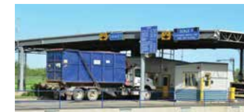
19 Weigh Scale The access point for all vehicles entering the EWMC.
