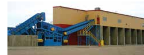
10 Construction & Demolition Recycling Facility (C&D) Processes mixed and segregated loads of wood, drywall, concrete, metals and asphalt shingles for recycling.
