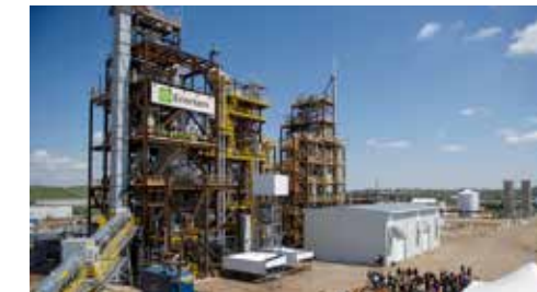
15 Waste to Biofuels & Chemicals Facility (Enerkem) Converts non-recyclable and non-compostable waste into methanol and ethanol.
