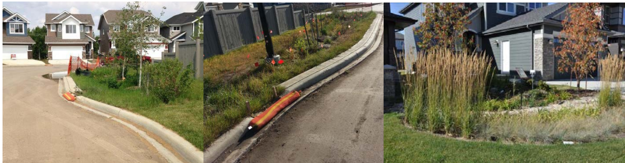
Big Lake Starling Road Bump Outs Bioretention in Edmonton AB. Photo by Xiangfei Li, City of Edmonton, 2013
