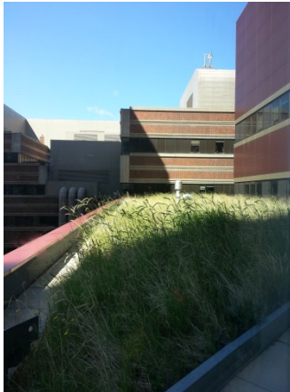
Green roof planted with grasses at the Mazankowski Heart Institute in Edmonton. The Institute has four extensive green roofs, with one visible from the Healing Garden. Photo by Xiangfei Li, City of Edmonton, 2013.
