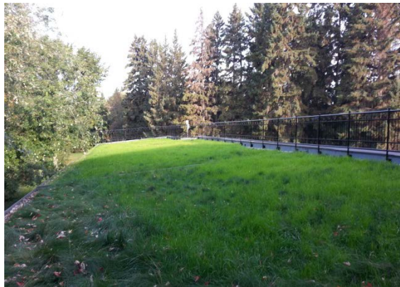
Victoria Golf Course Maintenance Building Green Roof in Edmonton, AB. Photo by Kenneth Yip, City of Edmonton 2014
