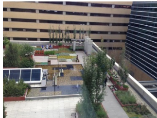
Intensive green roof at Lois Hole Alexandra Hospital, Edmonton, Alberta. Photo by Xiangfei Li, City of Edmonton, 2013.
