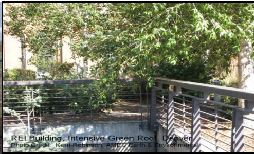
REI Building (intensive green roof), Denver, CO. Photo courtesy Kerri Robinson, AMEC Earth & Environmental
