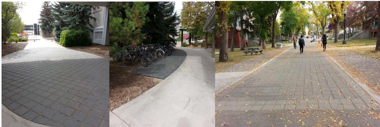
University of Alberta, Maintenance Building Walkway Permeable Pavers in Edmonton, AB. Photo by Kenneth Yip, City of Edmonton, 2014.
