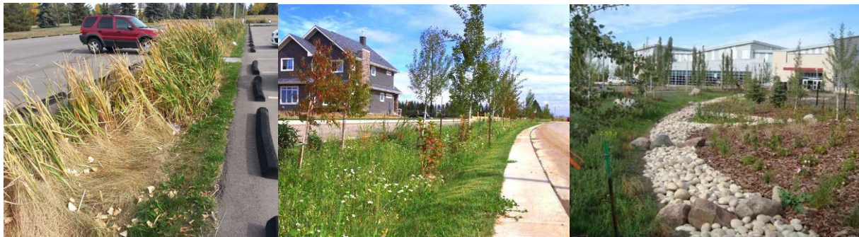
Bioswale at Mill Woods Parking Parking in Edmonton, AB to treat parking lot runoff. Photo by Kenneth Yip, City of Edmonton, 2014.
