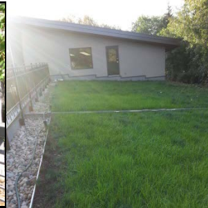
Victoria Golf Course Maintenance Building Green Roof in Edmonton, AB. Photo by Kenneth Yip, City of Edmonton 2014
