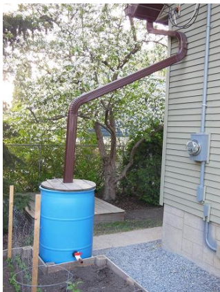
Residential rain barrel to harvest roof runoff for irrigating plants. Photo by Diane Wirtz, City of Edmonton
