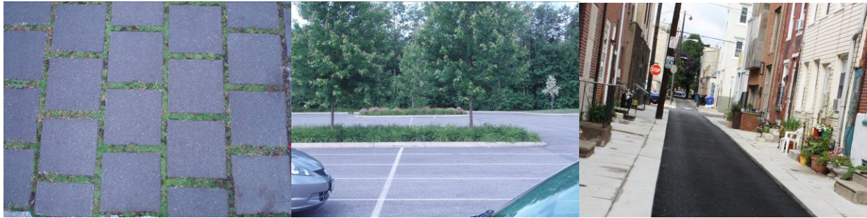
Pervious paver in Surrey, BC. Photo by Fayi Zhou, City of Edmonton, 2011
