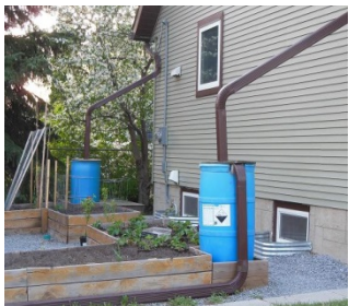
Residential rain barrel to harvest roof runoff for irrigating plants. Photo by Diane Wirtz, City of Edmonton
