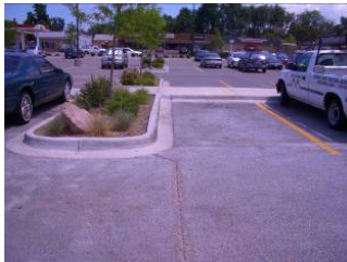
Porous Asphalt Parking Lot, Denver
