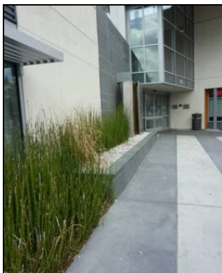
Flow through box planter, South Bay, CA. Photo Credit: Kerri Robinson, AMEC.
