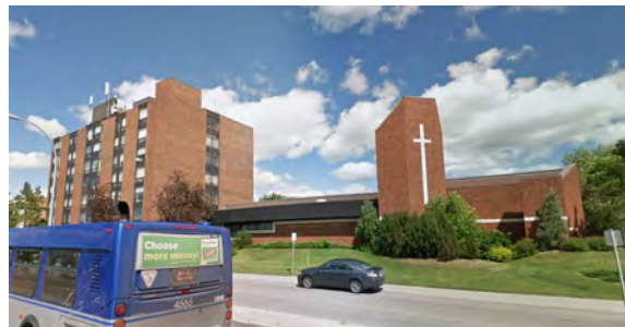
Ascension Church & Good Samaritan Place on the eastern boundary of the Plan Area
