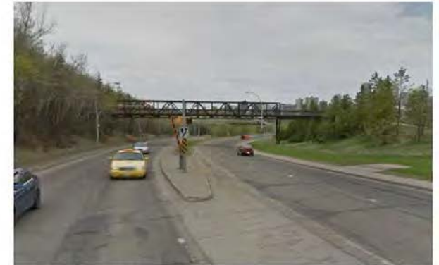
Existing Conditions (Looking west)
