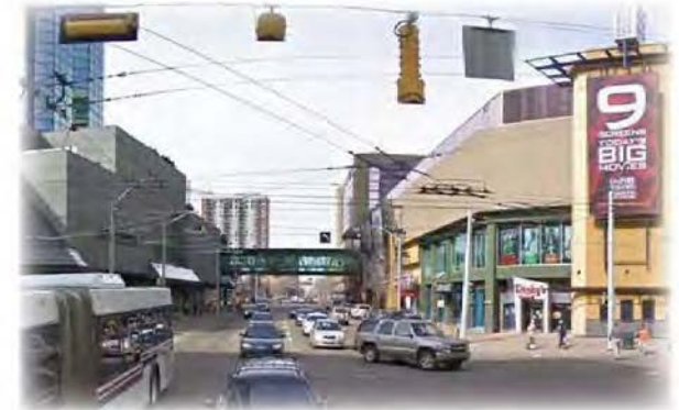
Existing Conditions (Looking west)
