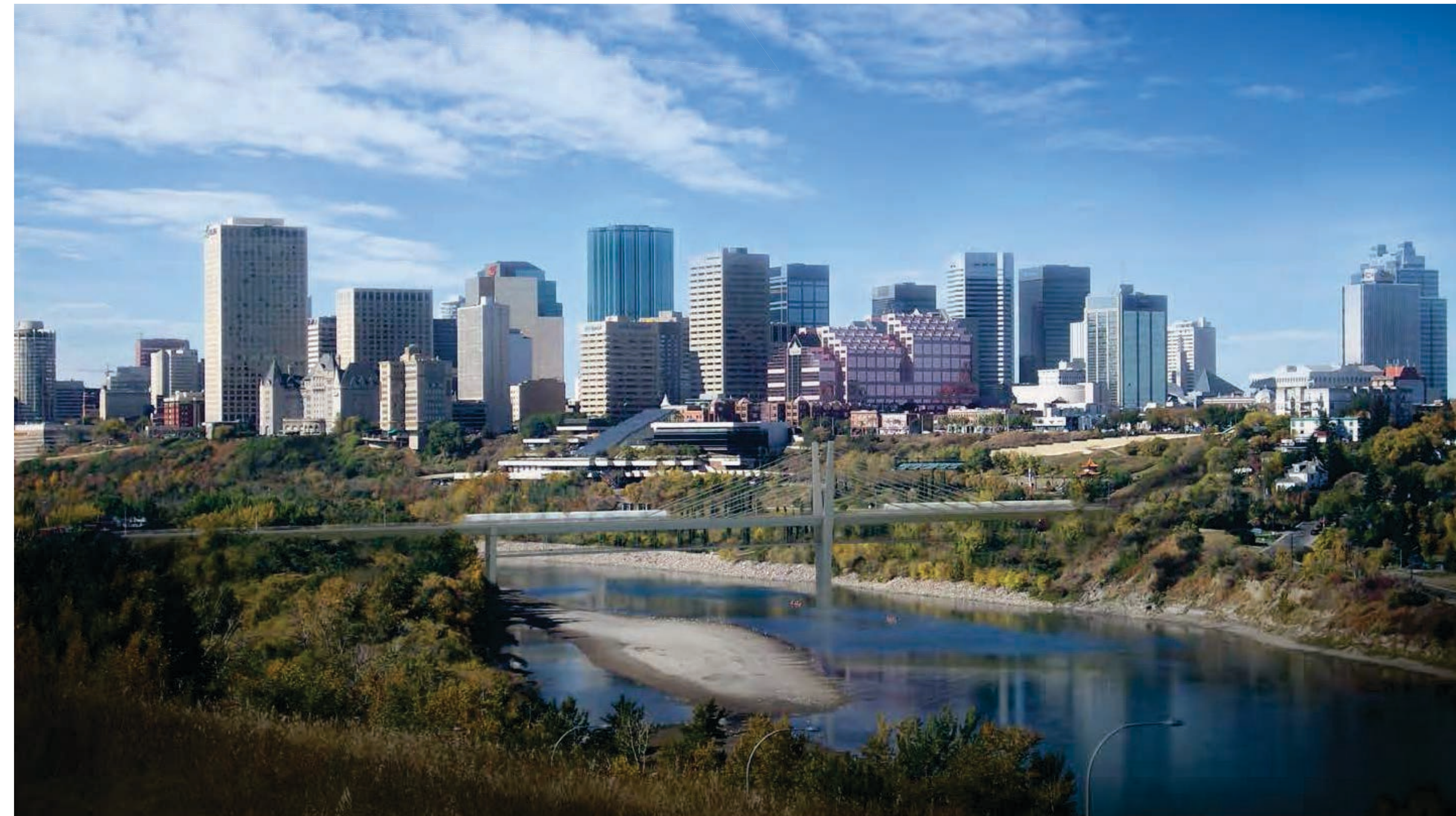
Extradosed bridge looking Northwest
