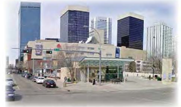
Existing Conditions (Looking west)
