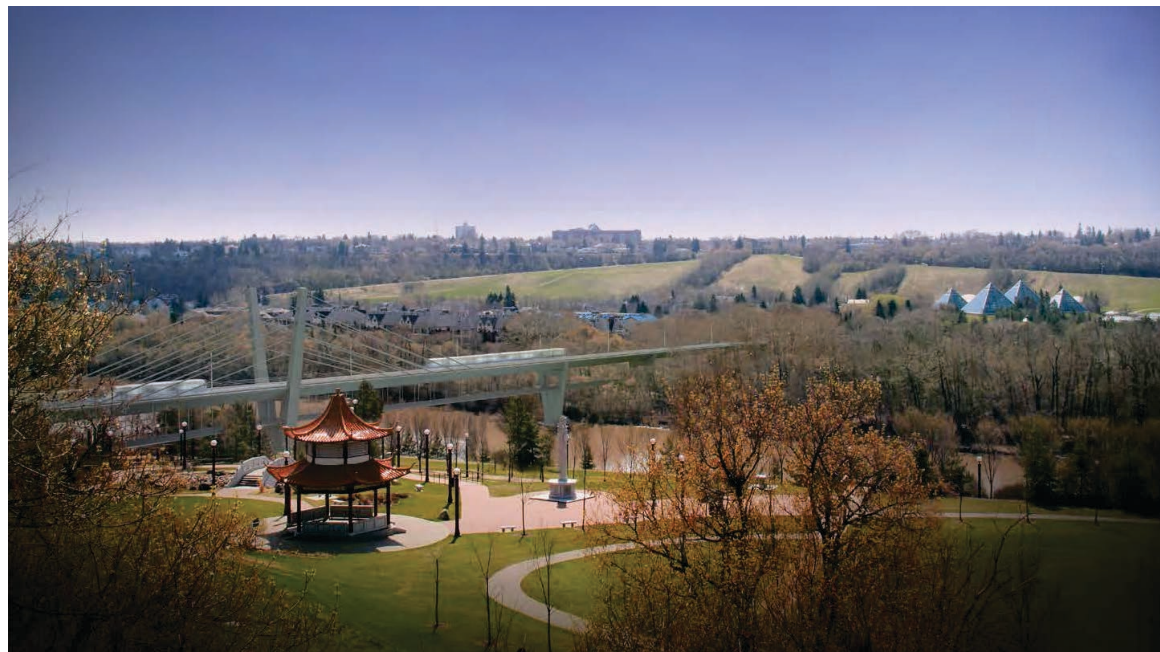
Extradosed bridge looking Southeast
