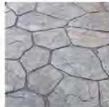
Paving (Patterned Concrete)
