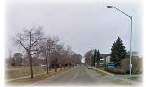
Existing Conditions (Looking west)
