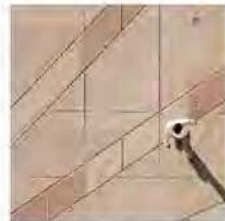
Paving (Patterned Concrete)
