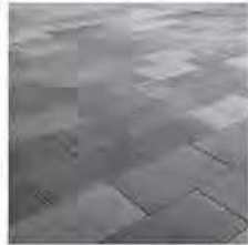
Paving (Patterned Concrete)
