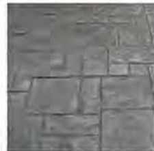
Paving (Patterned Concrete)
