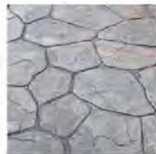
Paving (Patterned Concrete)
