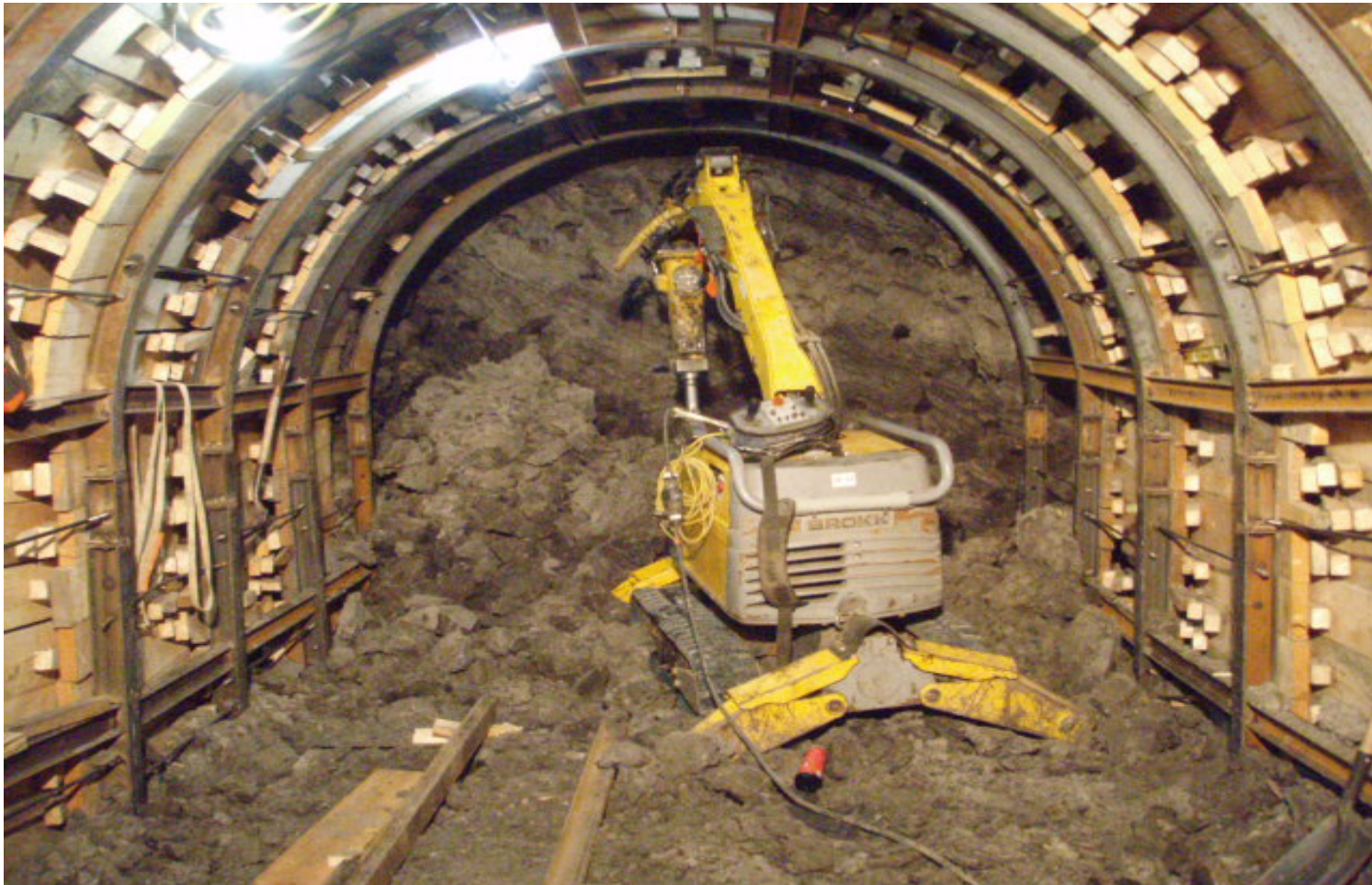
Figure 1c. WESS Stage W13 – Construction of undercut
