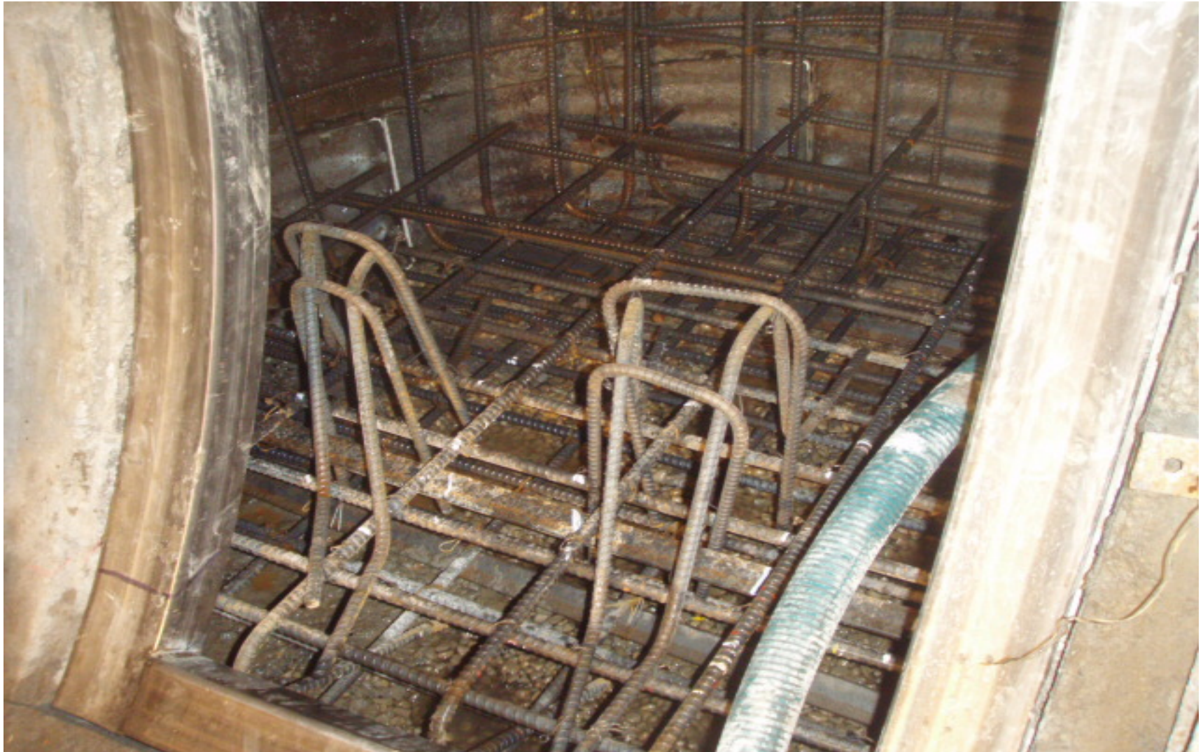
Figure 1b. NEST Reinforcing bars for Drop Manhole
