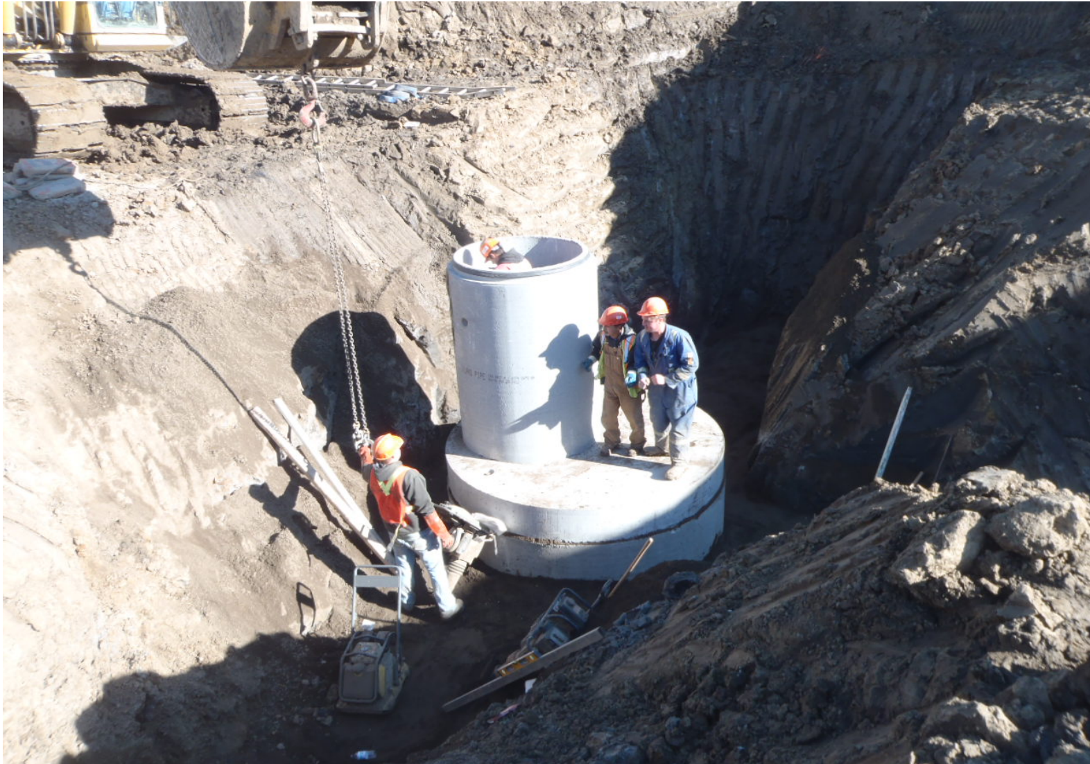
Figure 1d. SESS Stage SE4b – Construction Work
