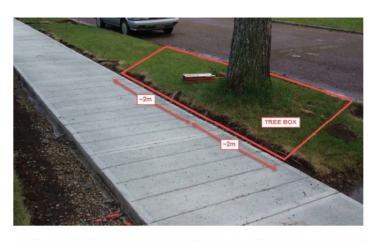
An area around each tree is maintained during construction to protect it and its roots
