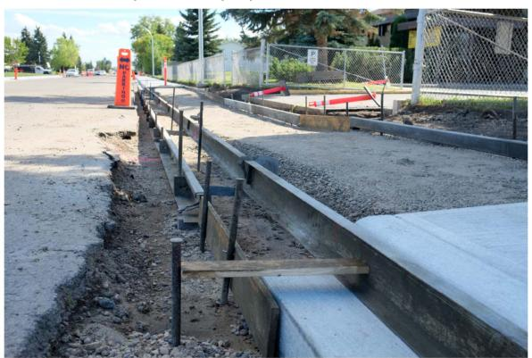
Forms are set in order to pour new concrete for the sidewalk.
