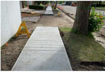
Extra deep cuts and rebar are added to the sidewalk to control where the sidewalk will crack and to keep the sidewalk intact as the tree's roots grow
