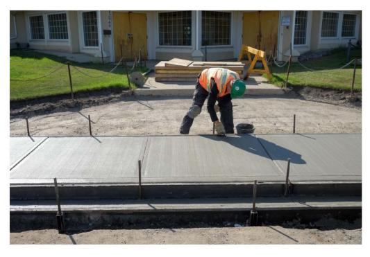
It takes approximately 3-4 weeks from the time concrete is removed to when it is cured and can be walked or driven on again.
