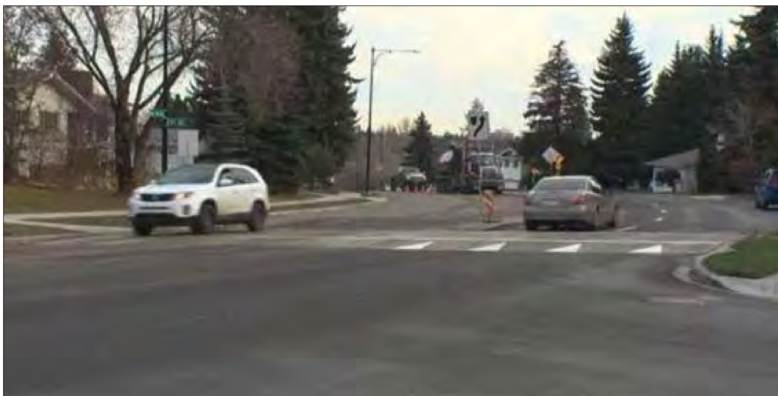
Raised crosswalk at Buena Vista Road and 85 Avenue
