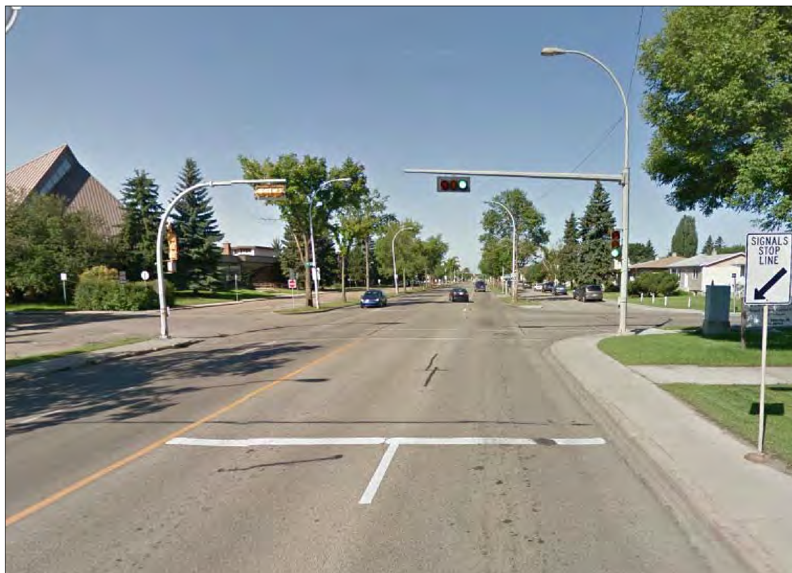
Pedestrian traffic signal on Whyte Avenue at 79 Street
