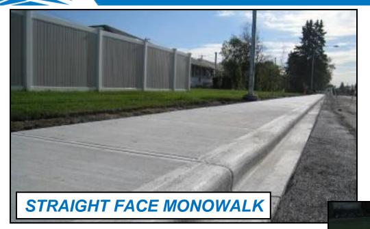
Local design constraints may cause curb and gutter type changes during construction to ensure positive surface drainage.
