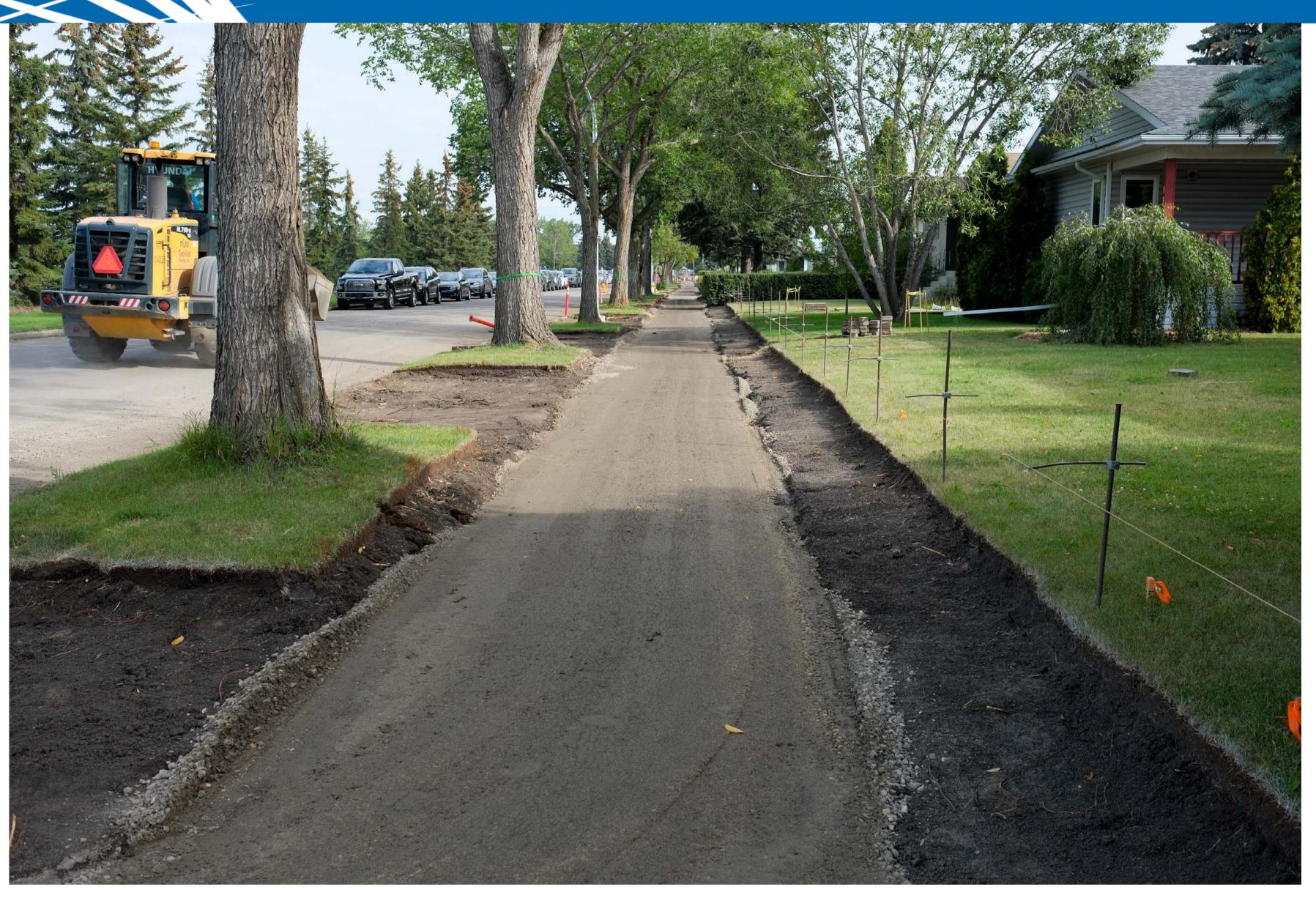
After removal of the existing sidewalk, gravel is placed and compacted to prepare for construction.
