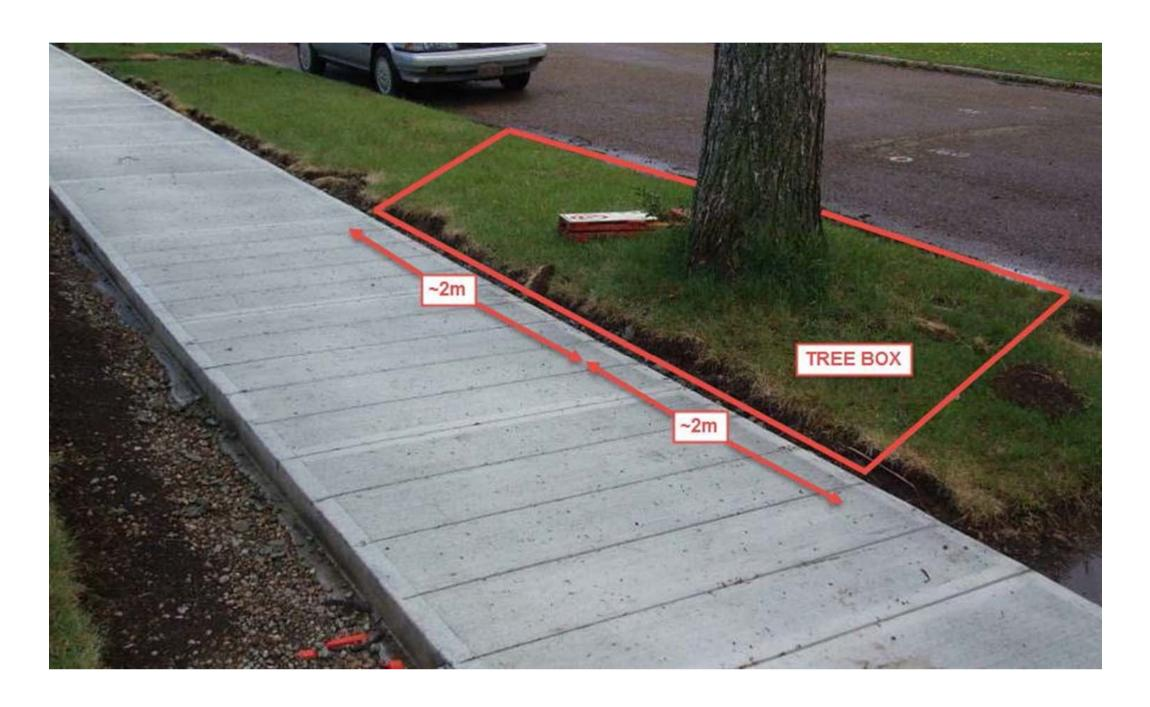
An area around each tree is maintained during construction to protect it and its roots
