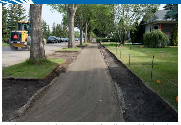
After removal of the existing sidewalk, gravel is placed and compacted to prepare for construction.
