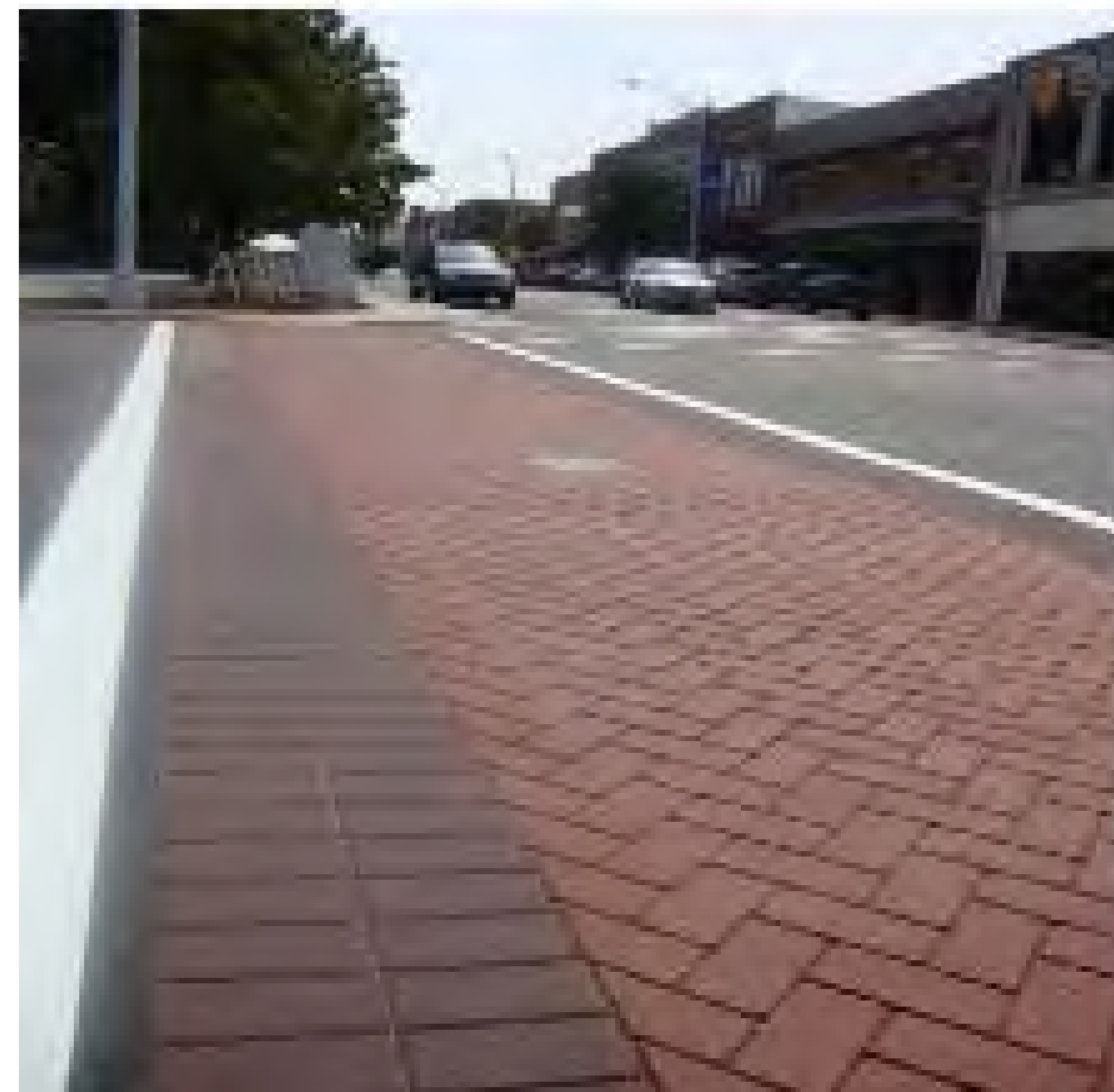
Stamped Asphalt Crosswalk
