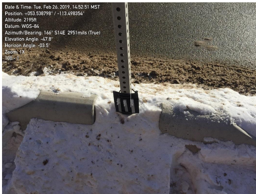
Figure 8 - Coupon Installed on Bicycle Lane Signpost
