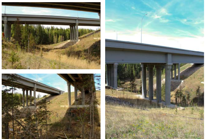
Figure 4.3: Wildlife crossing at Wedgewood Ravine and Anthony Henday. Note the high openness, gently sloped sidewalls, and incorporation of natural substrate and vegetation. (Photo Credit: Meghan Chisholm, Stantec Consulting Ltd. Used with permission.)
