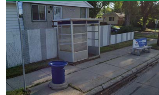
ETS bus stop at 121 Avenue and 46 Street with additional furnishings Figure 18
