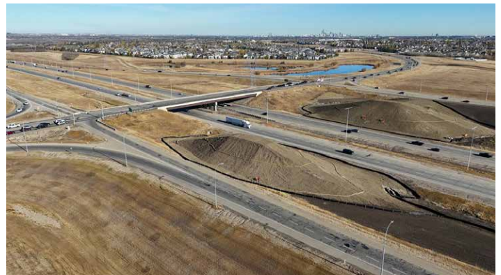
Stage Three site preparation 2025
