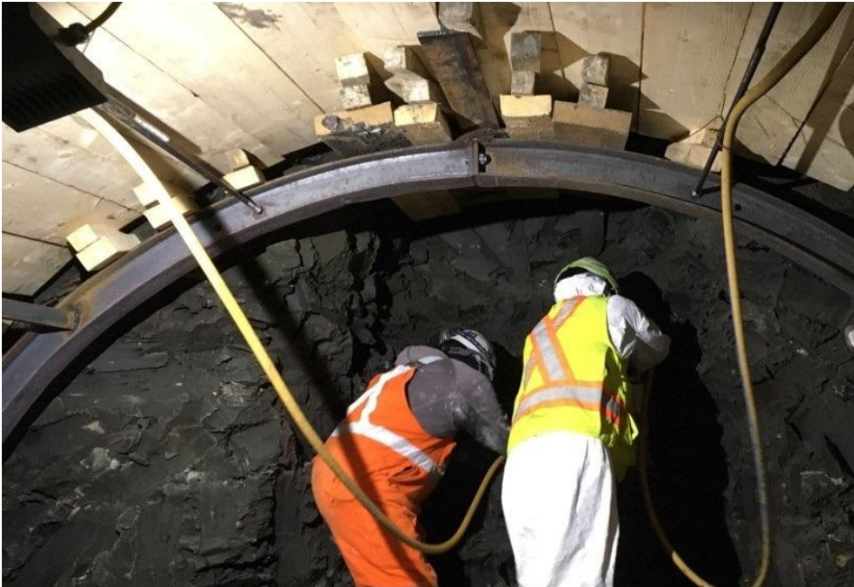
Figure 1a: NEST NC2/NC3, Undercut Excavation
