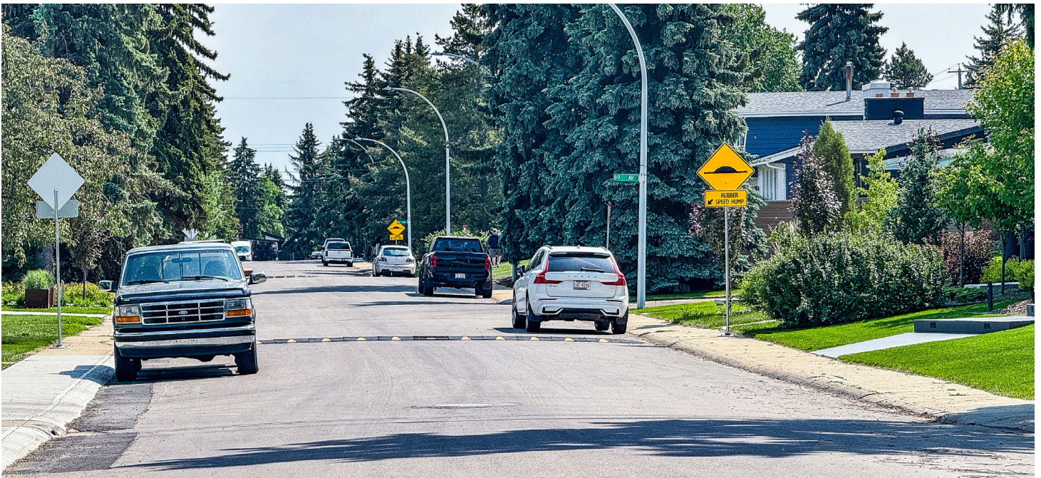
Temporary speed bumps were part of Edmonton's Street Lab on 140 Street
