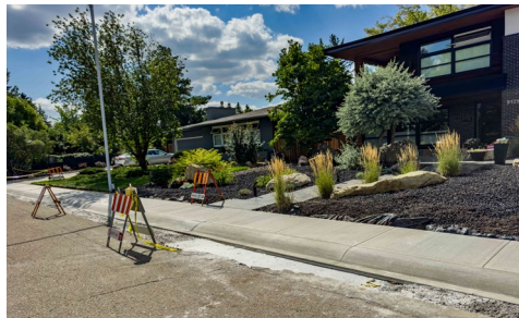
Sidewalk repairs on 141 Street
