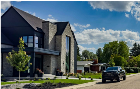
Residential infill on 141 Street
