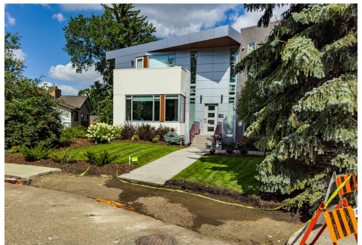
Development in the project area includes new infill homes (92 Avenue)
