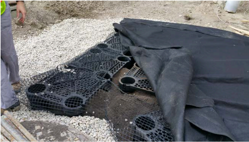
Soil Cell Installation
