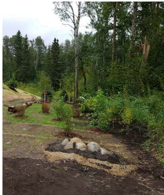
Ready Site (Outfall)
