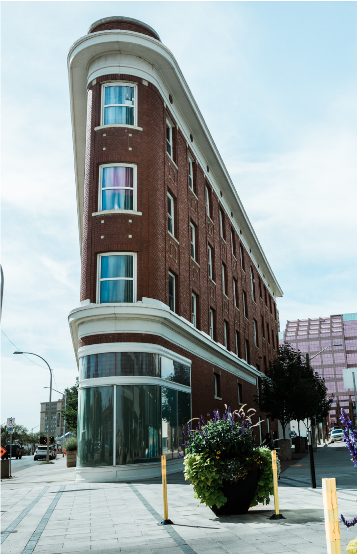
Gibson Block. City of Edmonton
