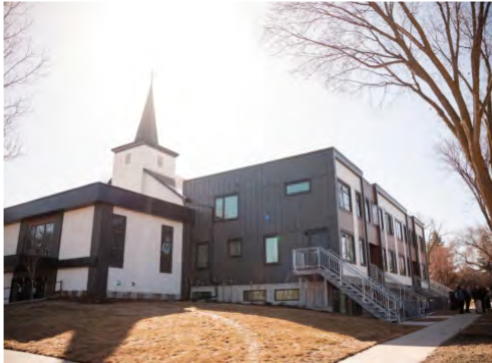
St. Paul's Lutheran Church redevelopment, King Edward Park with 11 affordable housing units.
