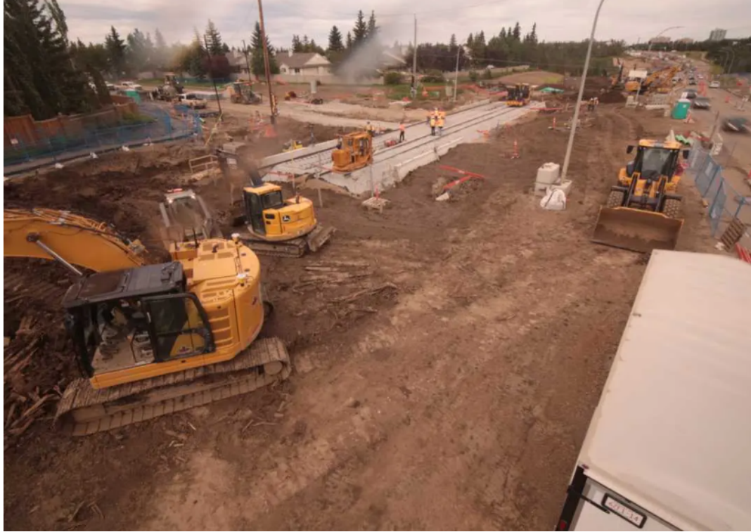
Screenshot from a timelapse video of Ledcor crews installing rail across the intersection (July 9, 2026)
