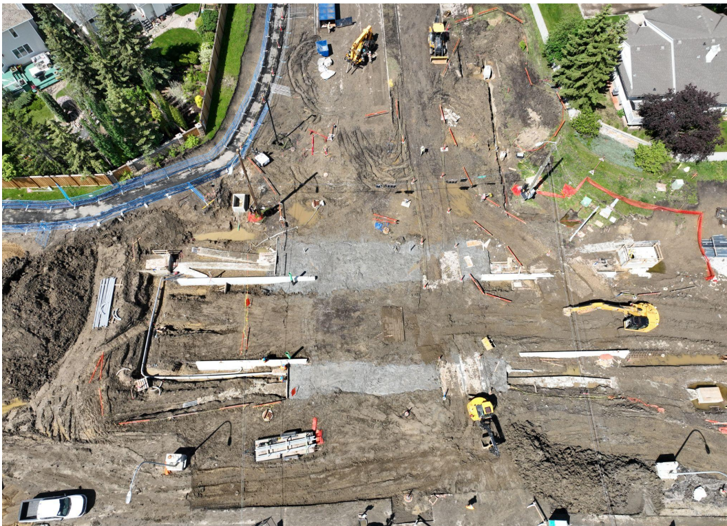
Aerial view of work zone at 12 Avenue west of 111 Street (June 2026)
