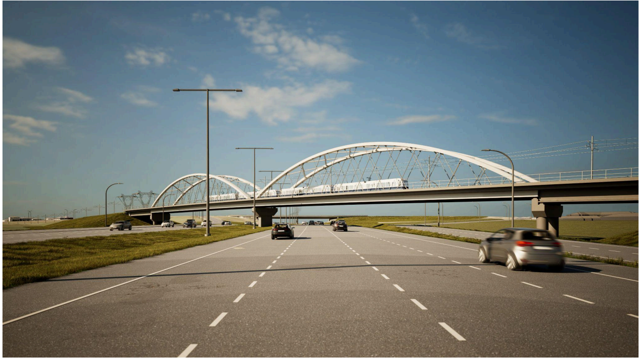
Anthony Henday Drive LRT Bridge (looking west)
