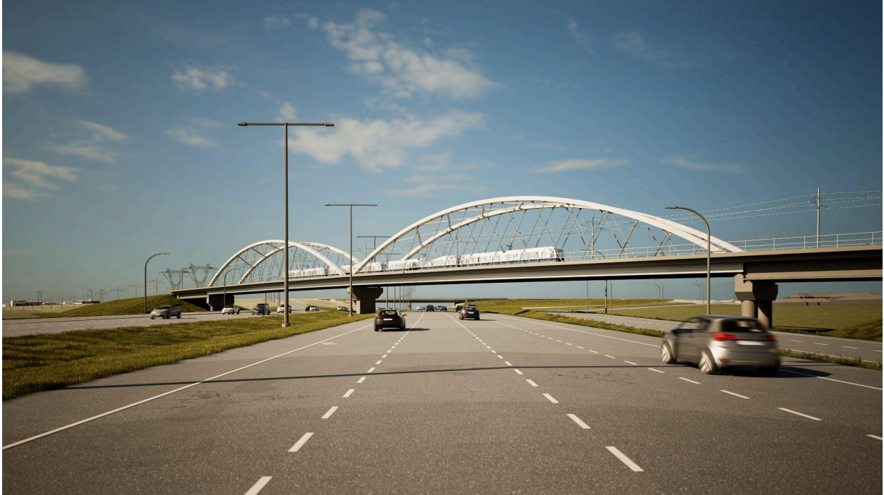
Anthony Henday Drive LRT Bridge (looking west)
