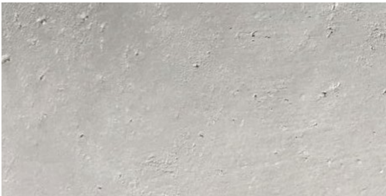
3 - ARCHITECTURAL FINISH CONCRETE
