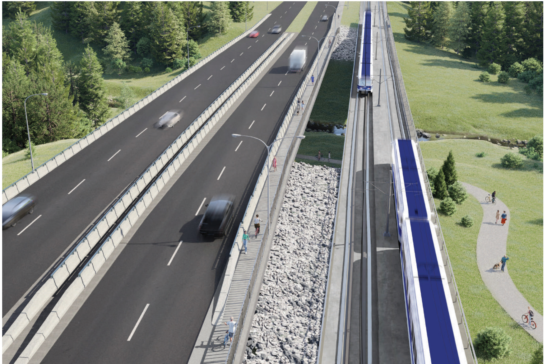
Blackmud Creek LRT bridge concept (looking south) with Shared-Use Path on the existing traffic bridge, and another path providing access to the ravine.
