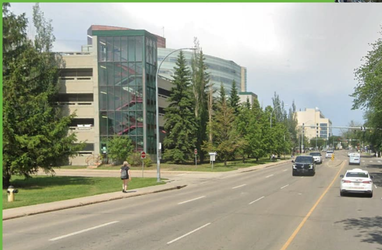
112 Street, Northbound view of multi-storey garage (Google Maps)
