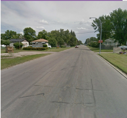
Figure 1 Missing sidewalks 119 Avenue between 49 Street & 50 Street
