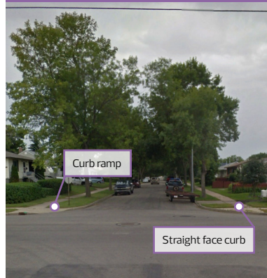
Figure 2 Intersection with straight face curbs and curb ramps 121 Avenue & 45 Street
