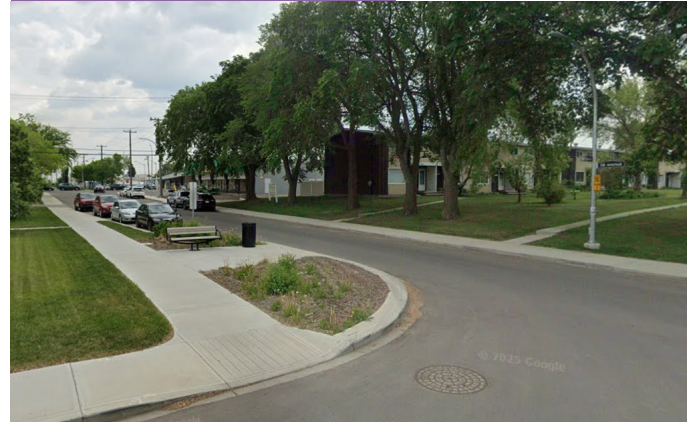
Figure 12 Curb extension example (Pleasantview)
