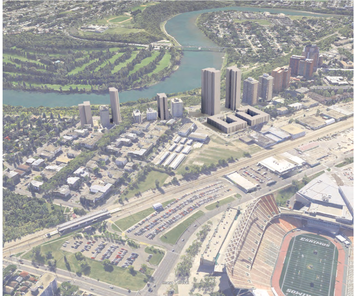
Figure 49: Stadium Station Plan Area—View to North Saskatchewan River (2012)
