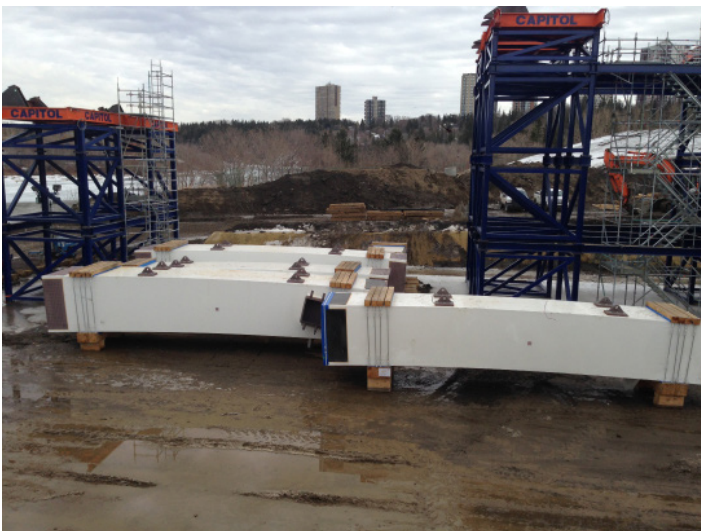
Central arch pieces in south side laydown area
