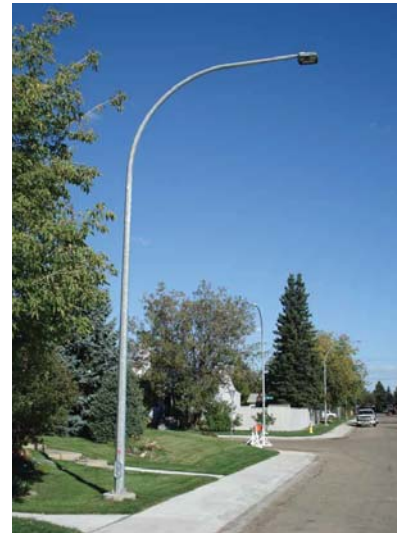
Standard galvanized street light
