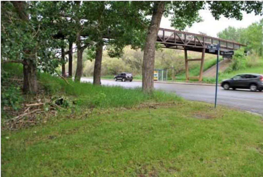
Plate 2.13: Lands extension for new tie-in trail, south of 98 Avenue, west of 96A Street, looking northwest (June 2014).
