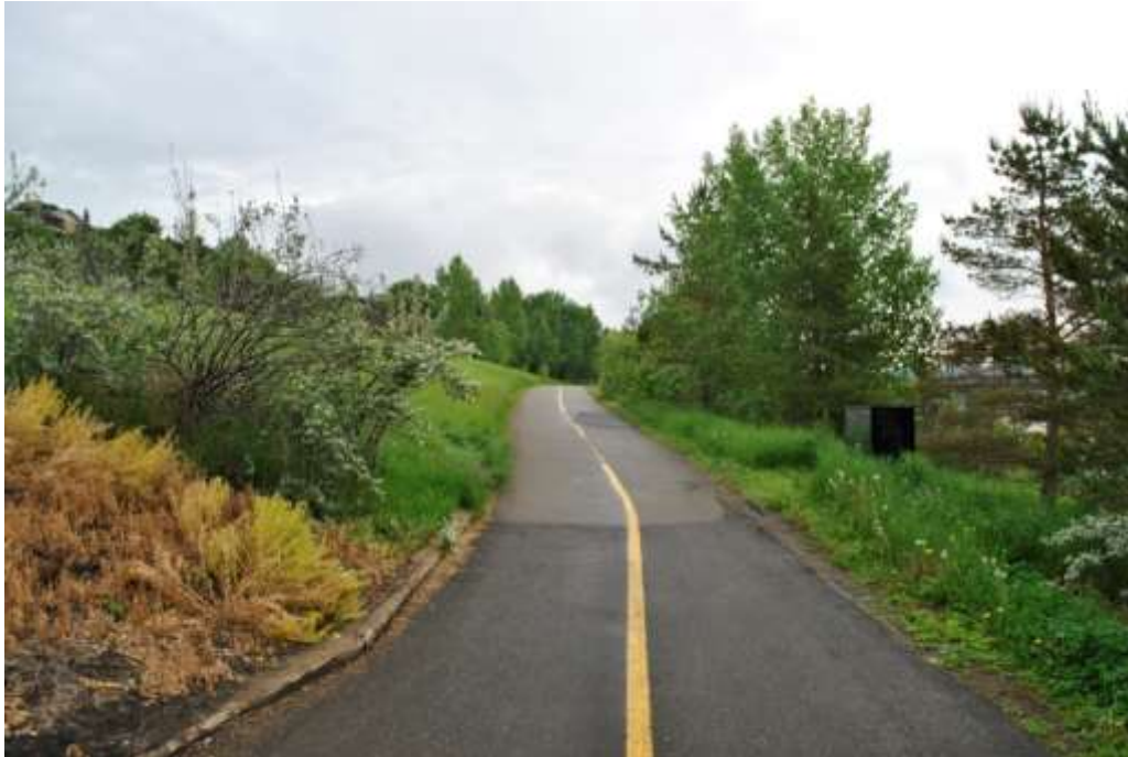
Plate 2.2: Trans Canada SUP to be used as Primary construction Access Route in LMRP.
