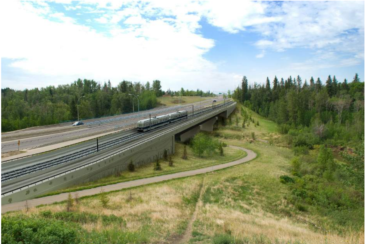
Bridge over Blackmud Creek looking south
