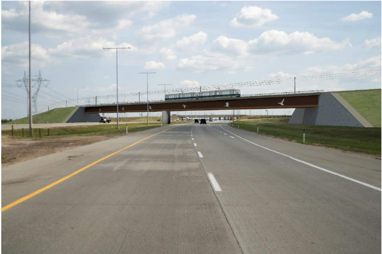
LRT Bridge over Anthony Henday Drive looking east
