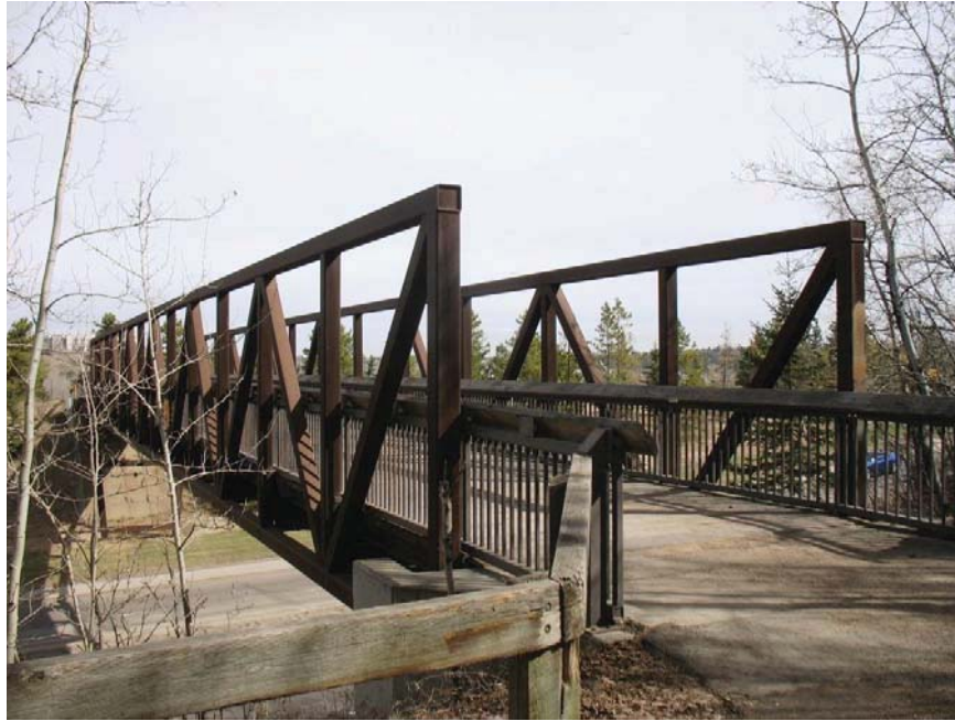
Plate 5.28. Connors Road pedestrian bridge
