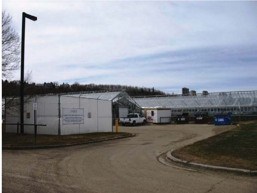
Plate 5.24. Staff parking and working greenhouses at the Muttart Conservatory
