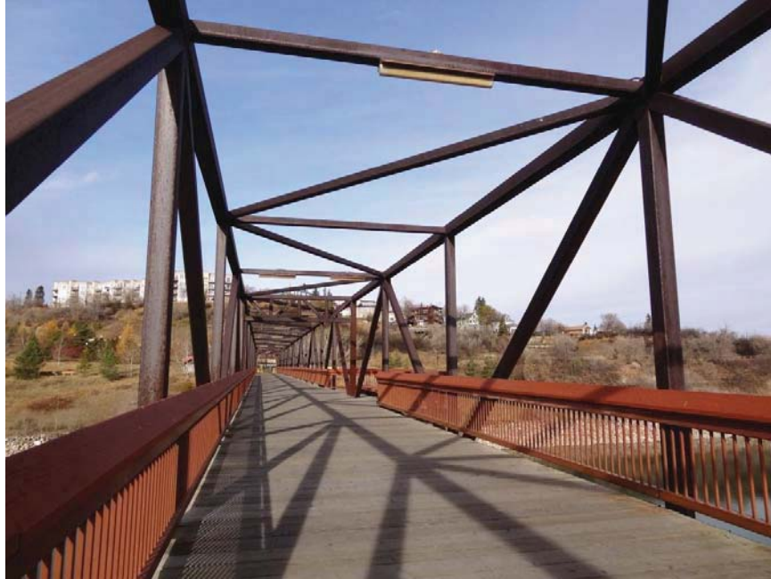
Plate 5.20. Cloverdale pedestrian bridge
