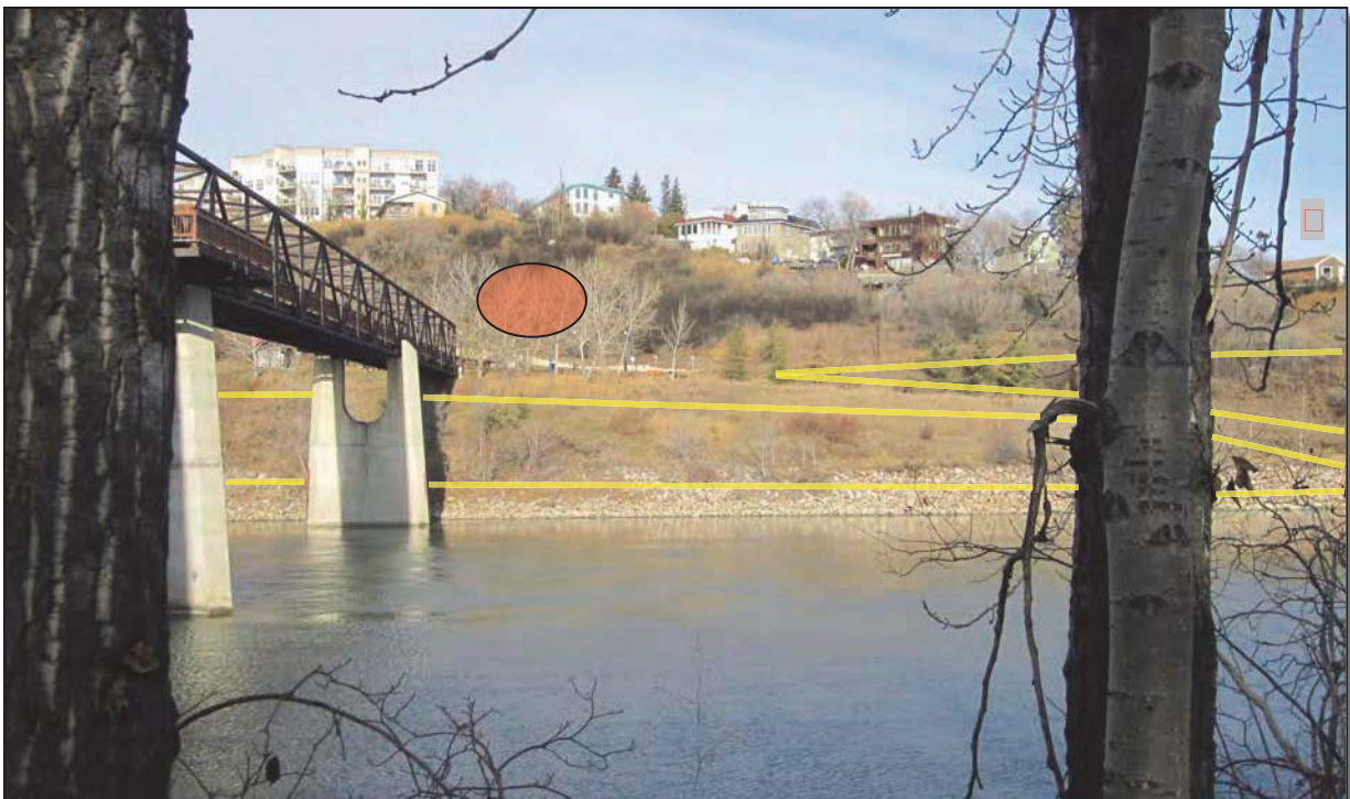
Figure 12. View facing north from south bank of North Saskatchewan River showing existing footbridge and approximate location of proposed LRT tunnel portal (●) on north valley slope. Note: bedrock likely near surface below thin vegetative/colluvial or landscaped cover (areas bounded by — lines). 1 = reference point (see house in Fig. 13)
