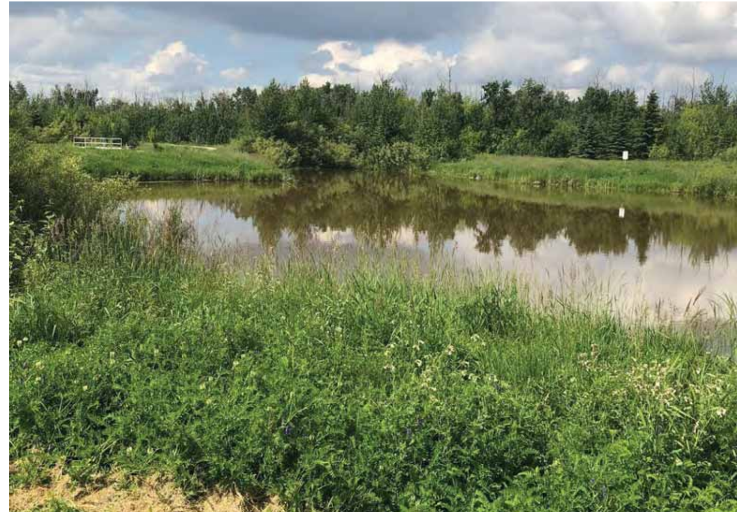
PYLYPOW STORMWATER TREATMENT WETLAND (AND KENNEDALE)
