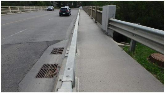
Plate 3. View east showing drainage CBs adjacent to southwest sidewalk on SPR.
