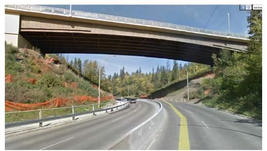
Plate 1. Existing single span steel-haunched girder bridge at 102 Ave over Groat Road.
