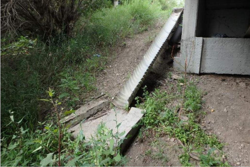
**Plate 4. View west showing overflow drainage infrastructure adjacent to southwest corner of SPR bridge abutment.**
