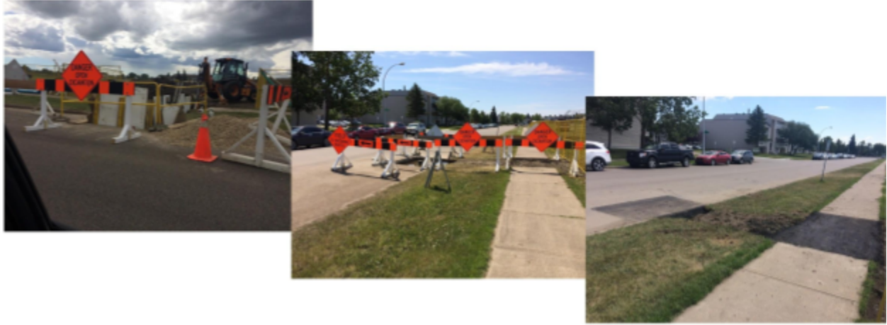
Figure 2: Site servicing connection work
