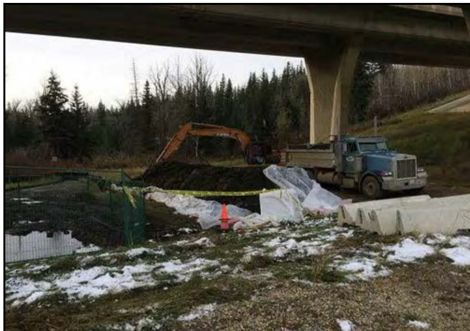
Photograph 6: The impacted soils were removed using tandem gravel trucks, and were hauled to the MCL Waste Systems Class II landfill near Leduc, Alberta (October 13, 2016).
