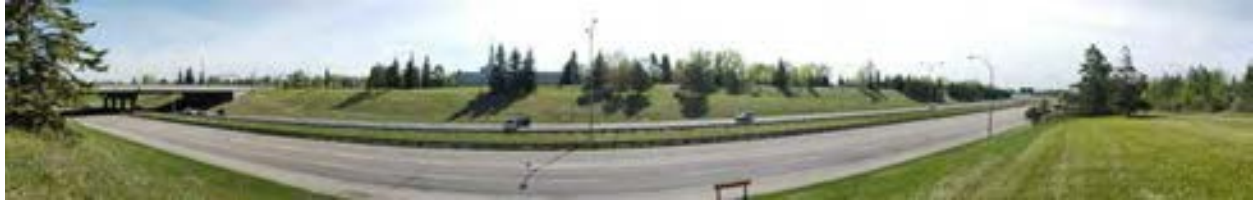
Figure 4. Panoramic view of Whitemud Drive, looking east. The overpass for 53 Ave can be seen on the left hand side of the image. Note heavily landscaped slopes and vegetation cover (erosion control measures) along the entirety of the freeway.
