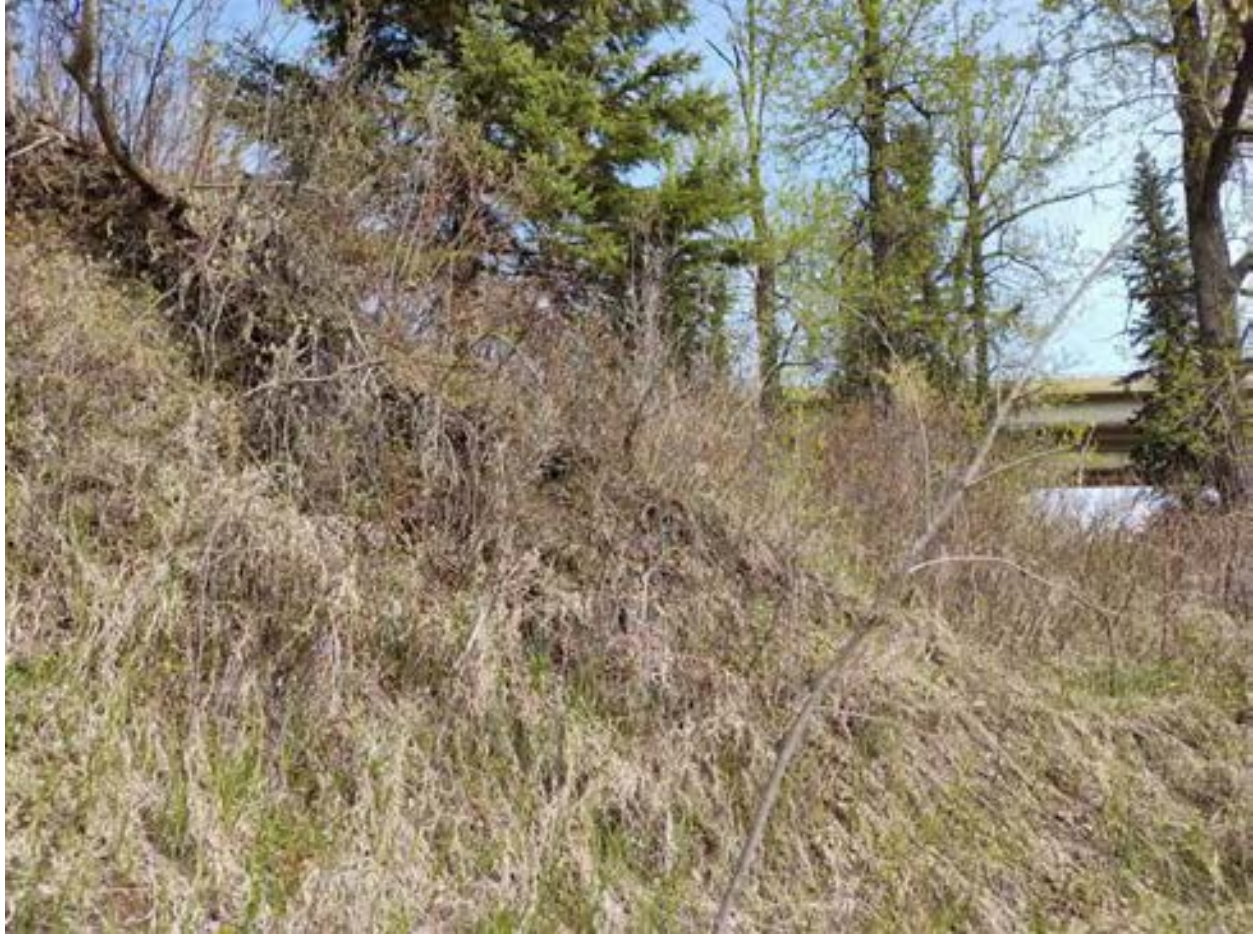
Figure 9. Small area of possible, highly weathered exposure. Note bridge deck at right of image. Photograph is taken looking north.
