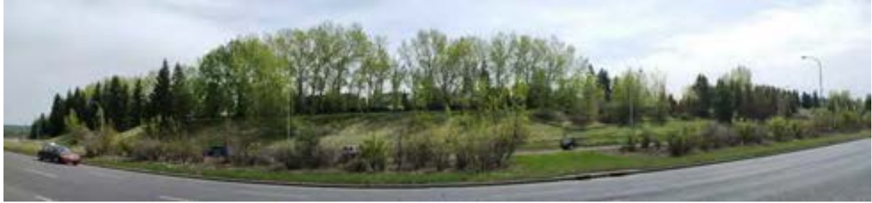
Figure 5. Panoramic view of Whitemud Drive looking east, near where the freeway begins to drop down into the North Saskatchewan River Valley. The river valley is towards the left of the image. Note heavy vegetation cover along the length of the freeway.
