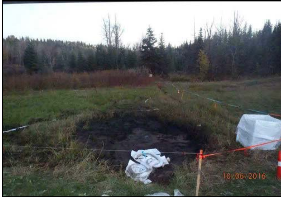
Photograph 1: Diesel staining, resulting from the MVA, beneath the drainage culvert on Whitemud Drive (October 6, 2016).
