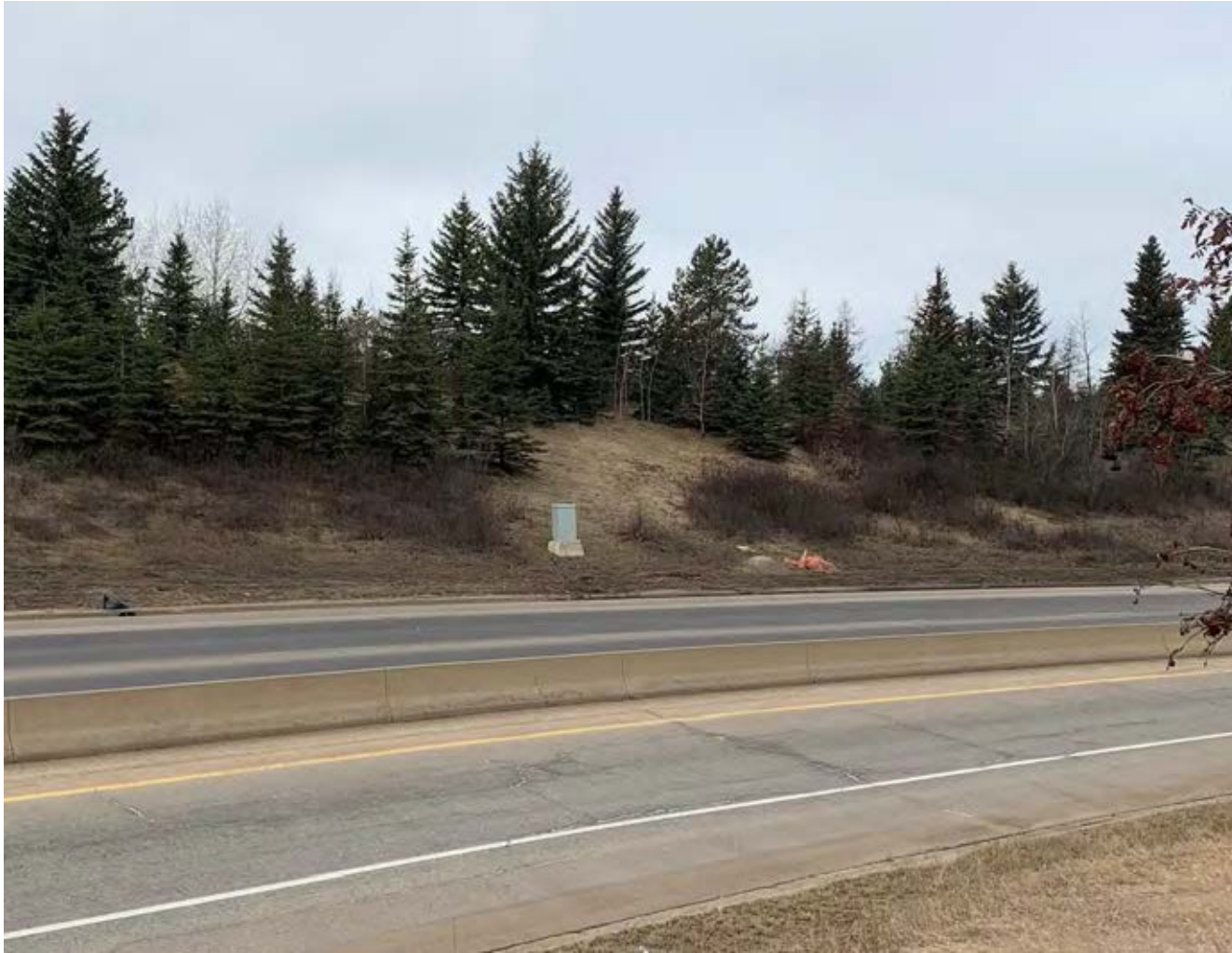
Photograph 5 – Facing southwest from WMD-Terwillegar Drive interchange, trash bag and debris along southbound WMD. April 22, 2020.
