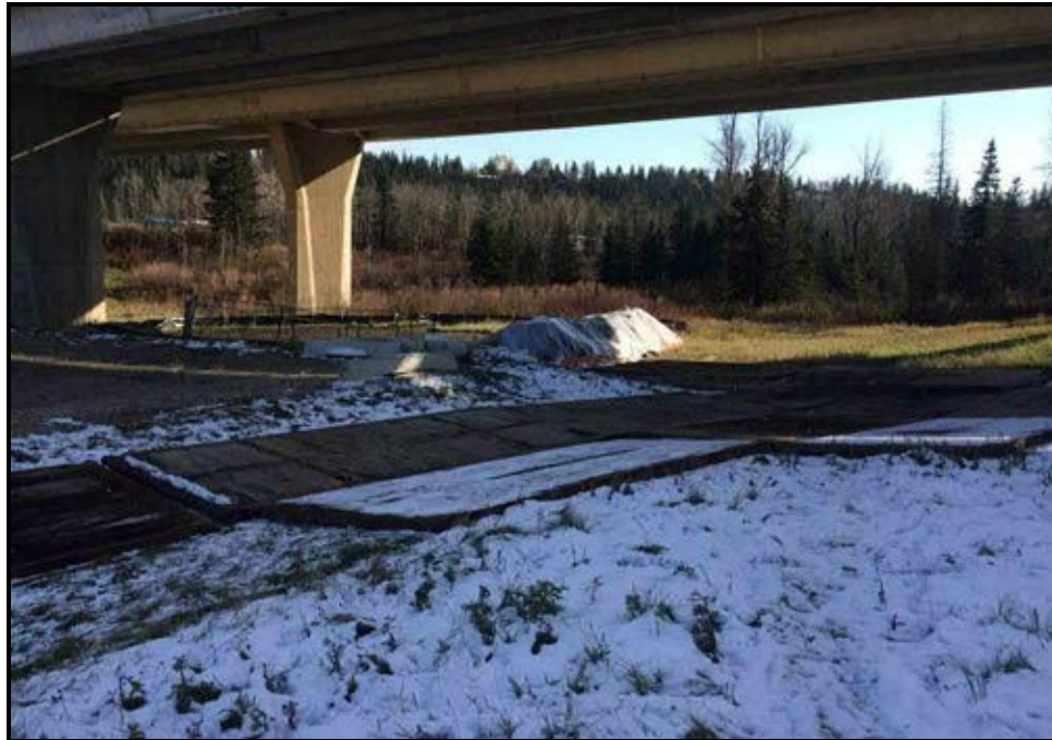
Photograph 5: Rig mats were installed from the gravel-surfaced parking lot to the Site, in order to provide access for loading of haul trucks and removal of the impacted soil (October 12, 2016).
