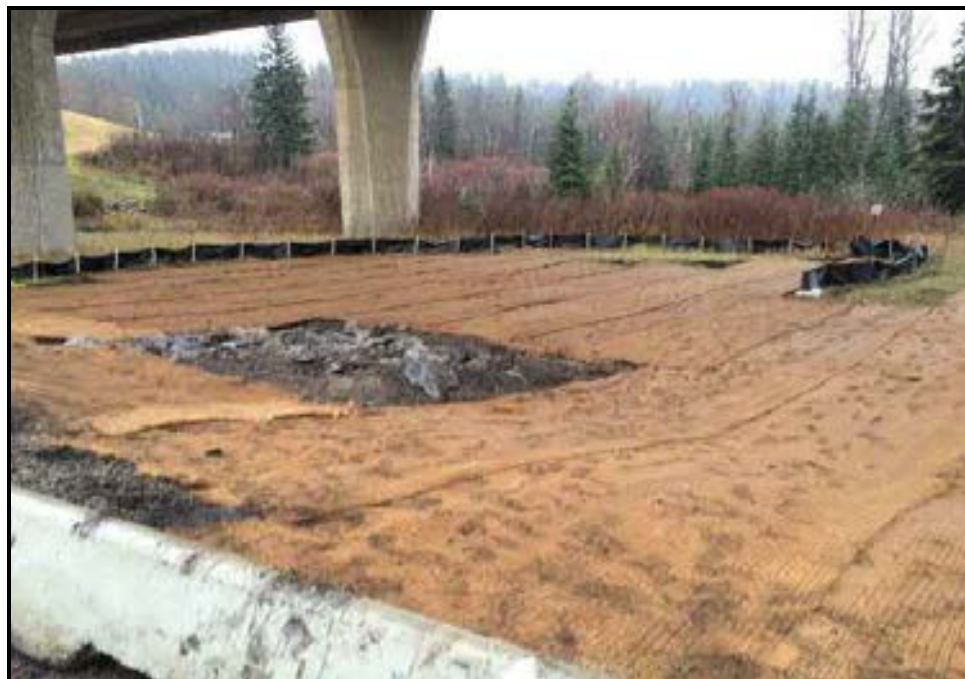
Photograph 10: The Site was re-seeded with a custom, native reclamation seed mix and then covered with erosion control blankets (October 25, 2016).
