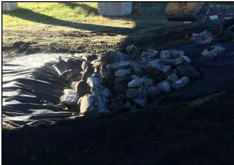
Photograph 8: The seepage pit was filled with rip rap (October 21, 2016).
