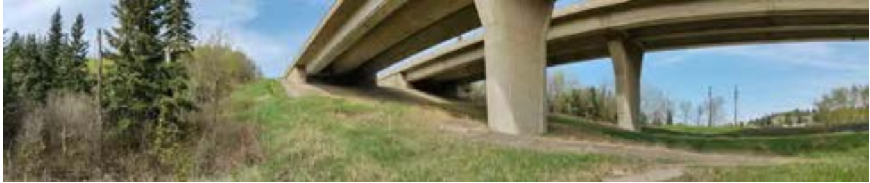
Figure 11. View from Whitemud Creek, looking northwest, of the slopes underneath the Rainbow Valley Bridges. Note the small patches of exposures in the centre of the image; these patches are all reworked deposits, likely from the original construction of the bridges.
