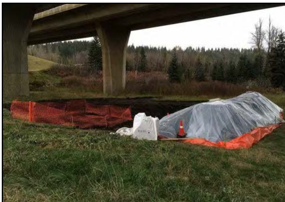
Photograph 4: Impacted soils were contained in a poly-lined cell onsite for future disposal once landfill approval was granted (October 7, 2016).
