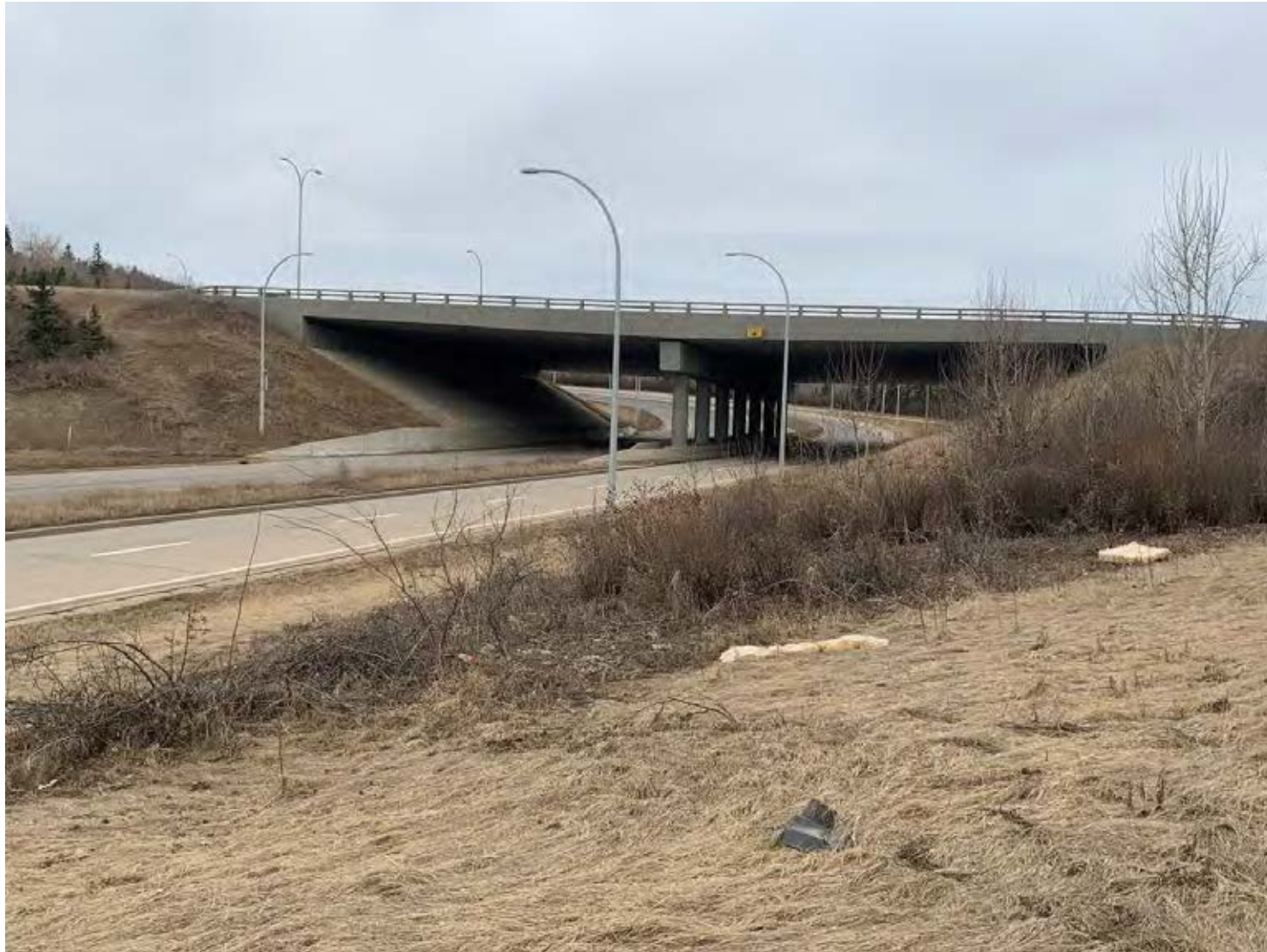
Photograph 2 – Facing southwest to WMD-Fox Drive interchange, debris along ramp. April 22, 2020.
