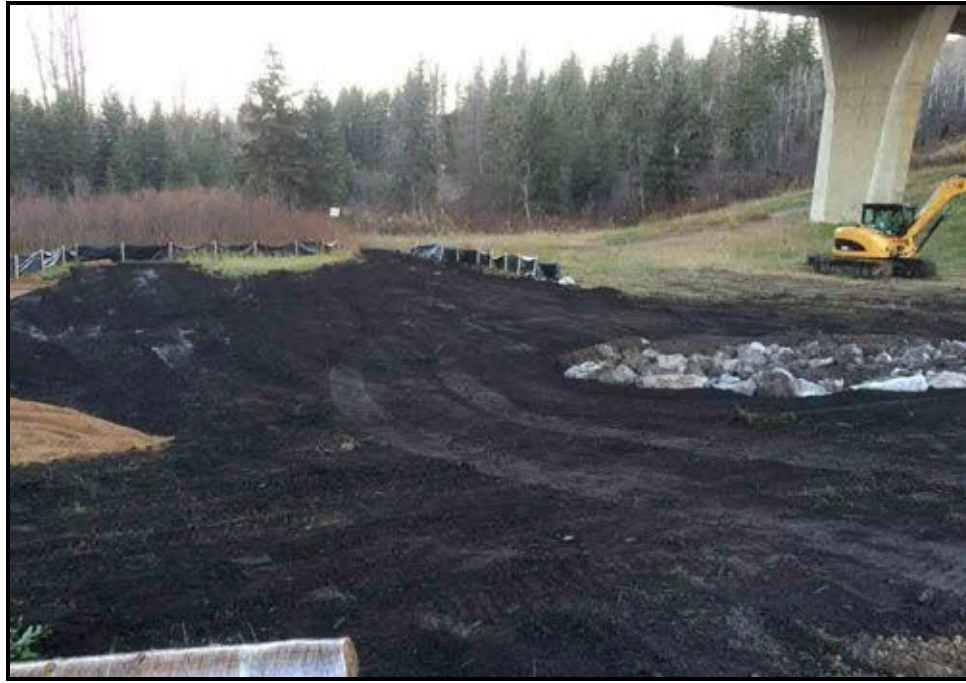
Photograph 9: The Site was backfilled with topsoil, re-contoured and track packed (October 21, 2016).
