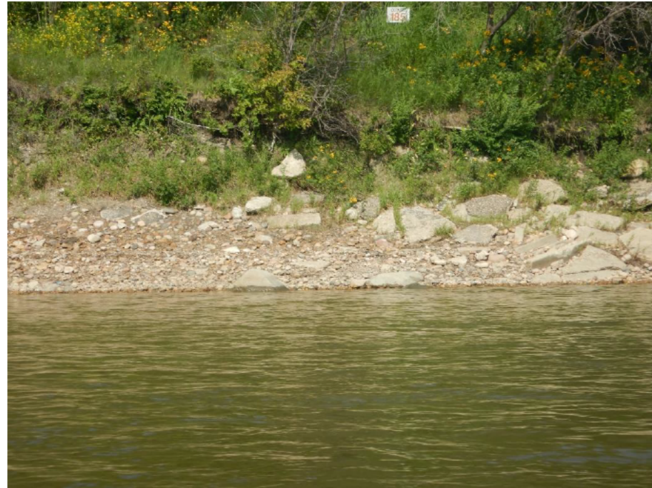
7) Looking at concrete bank armoring downstream of High Level Bridge.
