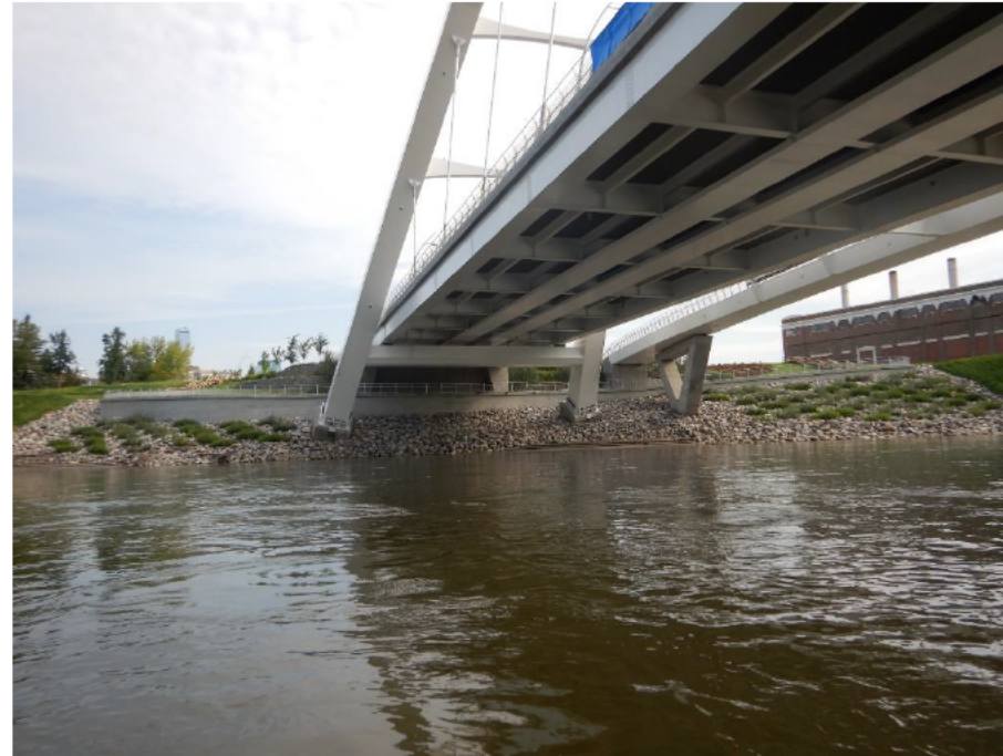
8) Looking at vegetated riprap on left bank at Walterdale Bridge.
