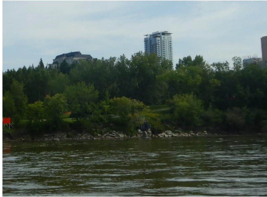
2) Looking at existing outfall on left bank upstream of Groat Road Bridge.
