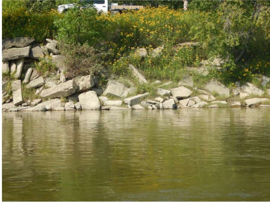
1) Looking at concrete bank armoring upstream of Groat Road Bridge.
