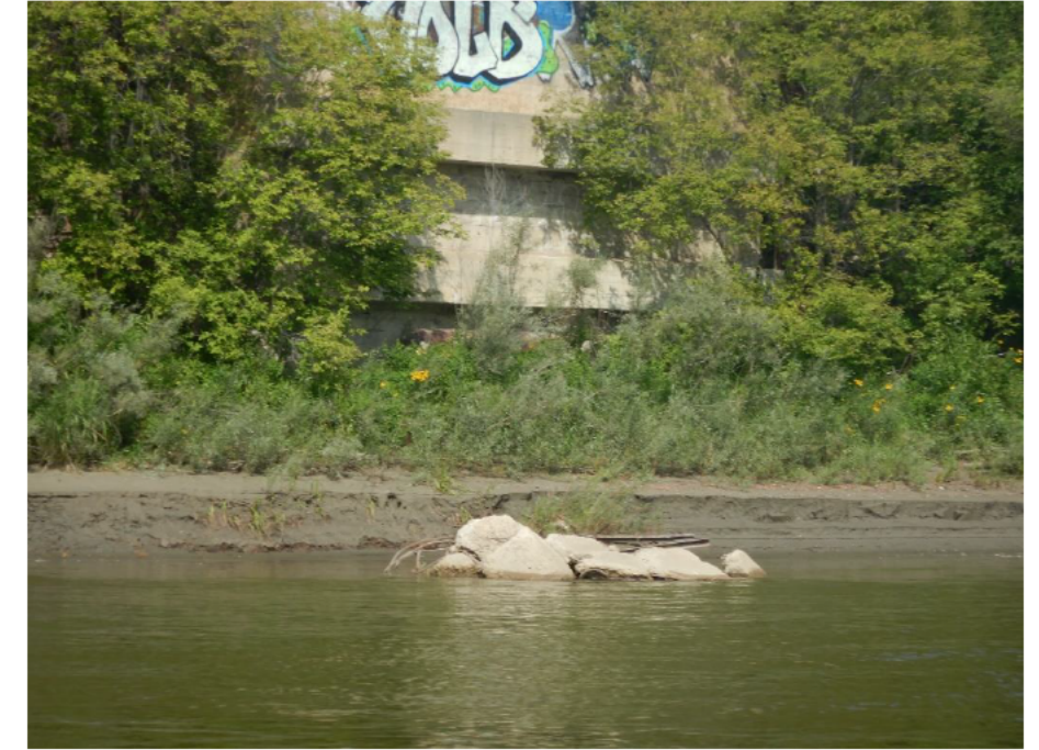
9) Looking at left bank downstream of Walterdale Bridge.
