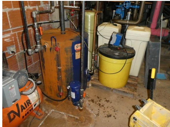
D3020.01.04 Water Treatment Equipment* (Steam Boilers)
