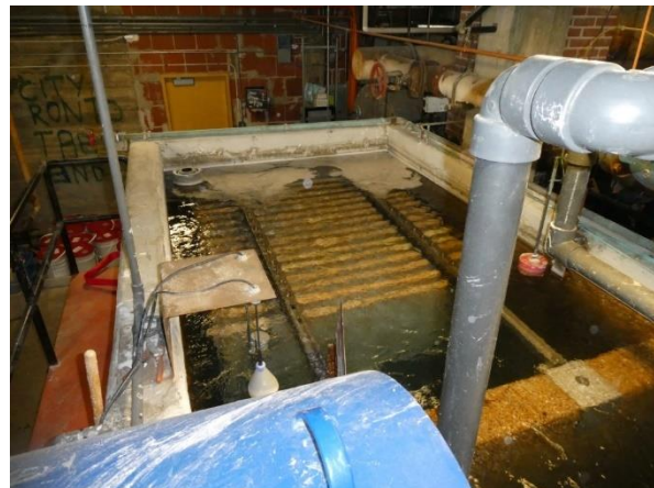
Aquatic Facilities* (Pool Filter Tank)
