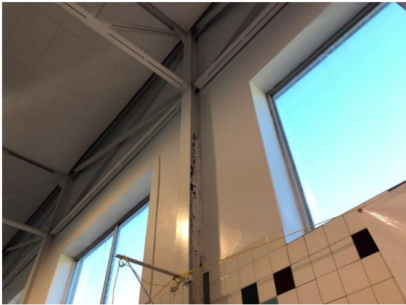
B1020.01.04.02 Steel Joists* Location: Pool area Component: Roof Structural Frame
