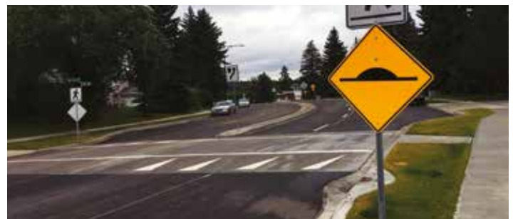
Example of a raised crosswalk
