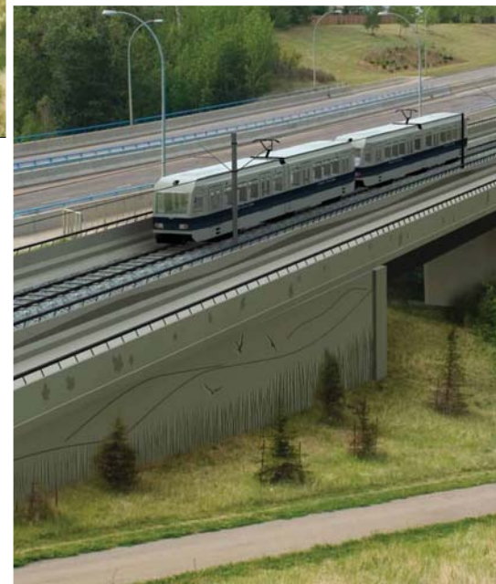
Blackmud Creek Bridge Close Up
