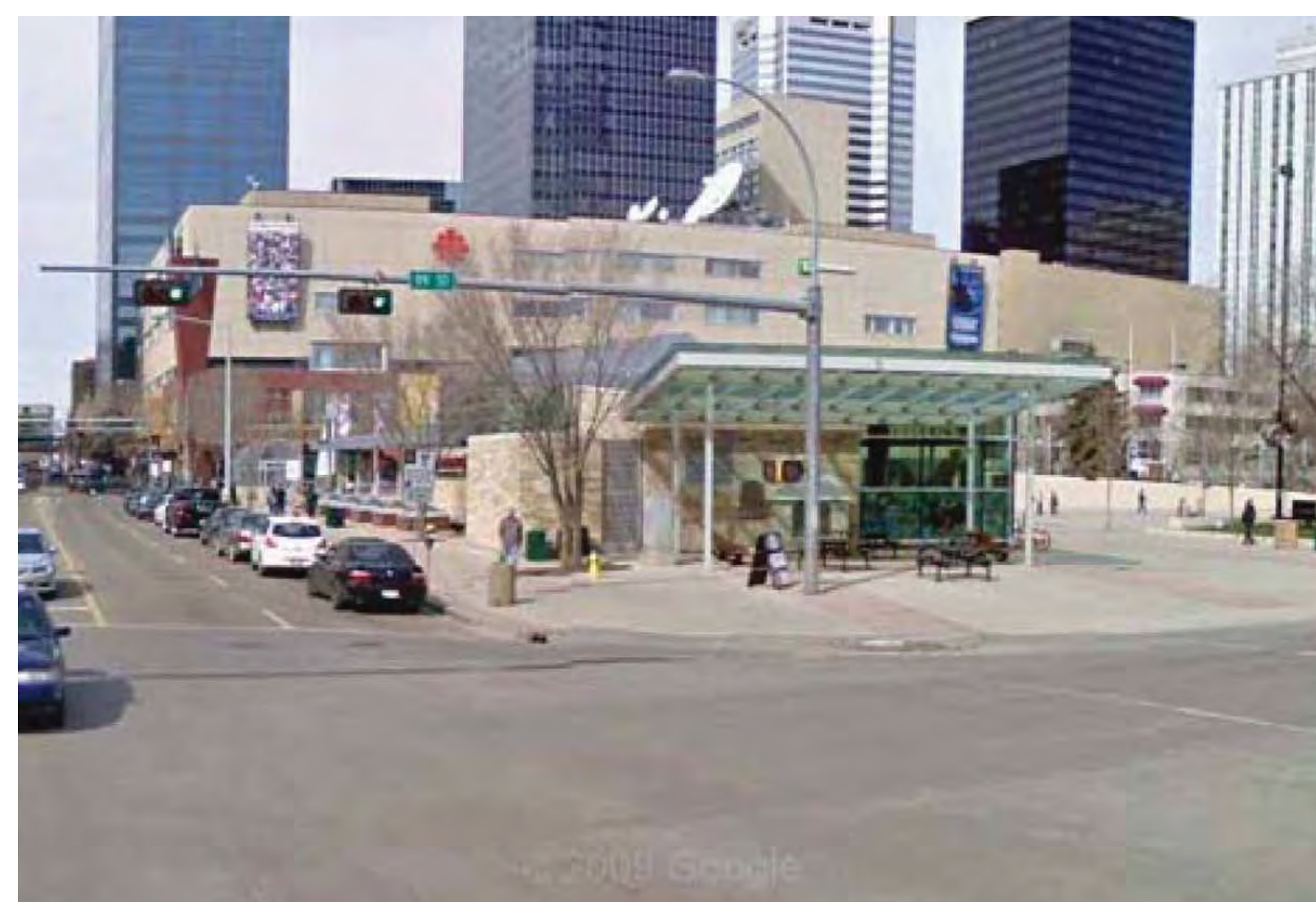
View A - Existing Condition
