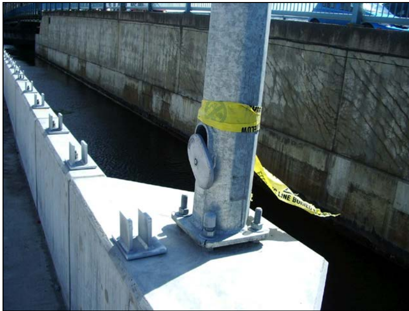
Figure 4 - Example Foundation on Bridge Structure
