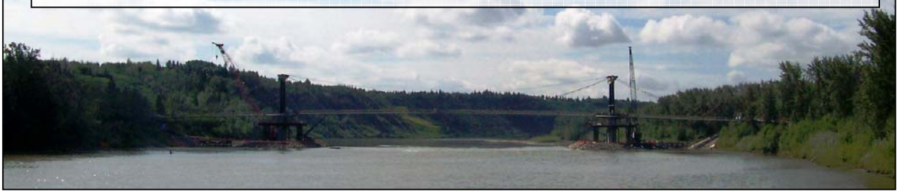
NORTH SASKATCHEWAN RIVER FORT EDMONTON FOOTBRIDGE - View from North
