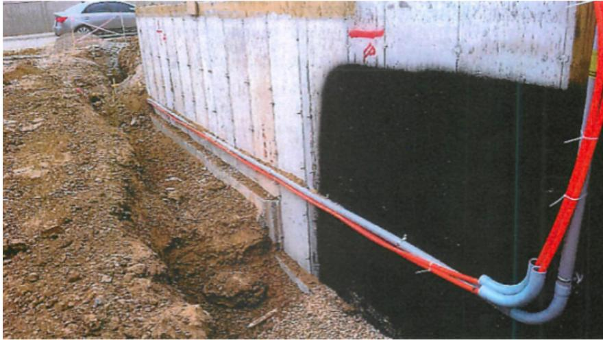
**Figure 3 |** Sample of Secondary Method: The conduit is correctly backfilled as it leaves the foundation
