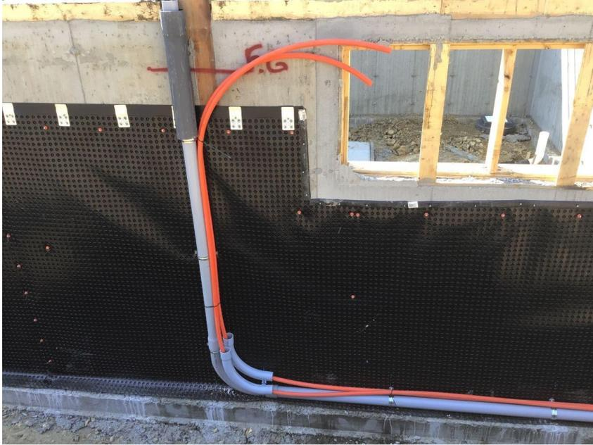
**Figure 1** | Sample of Primary Method: Clear view of the pipes and strapping placement.
