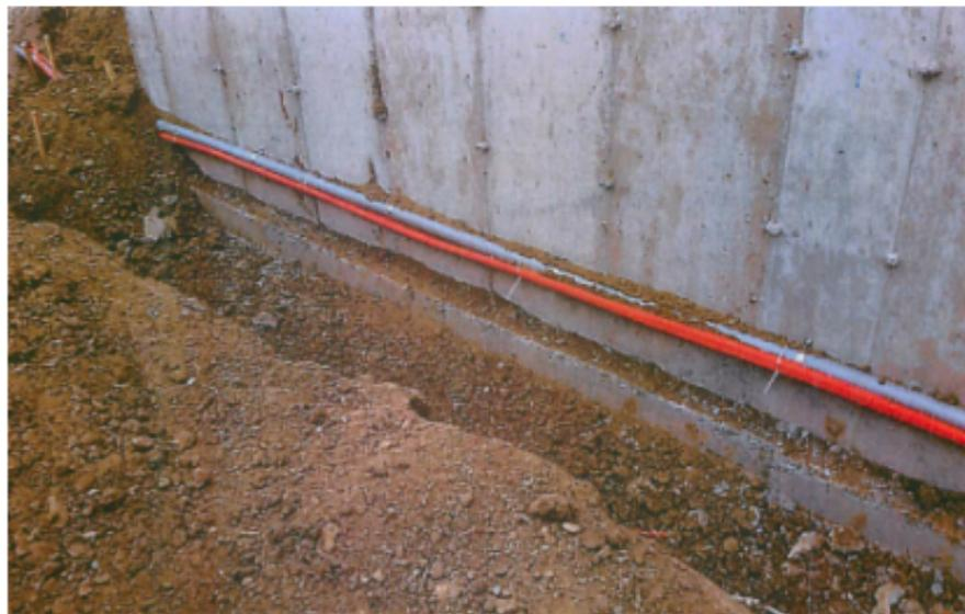
**Figure 4 |** Sample of Secondary Method: Top view of the conduit as it leaves the trench
