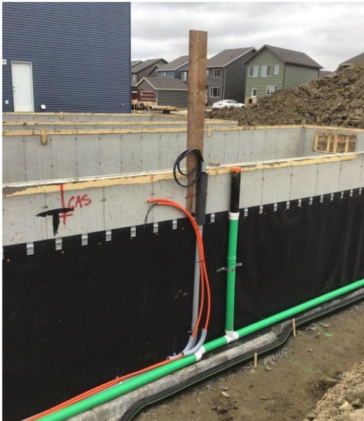
**Figure 2** | Sample of Primary Method: The horizontal conduit will have priority and will be installed tightly to the footing.
