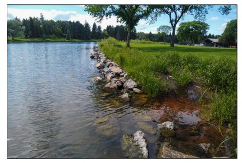
Figure 3. Hawrelak Lake east shore, with riprap and a narrow, unmowed strip of vegetation
