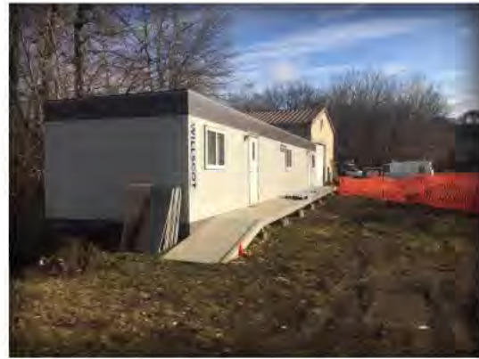
New trailer east of the office building.
