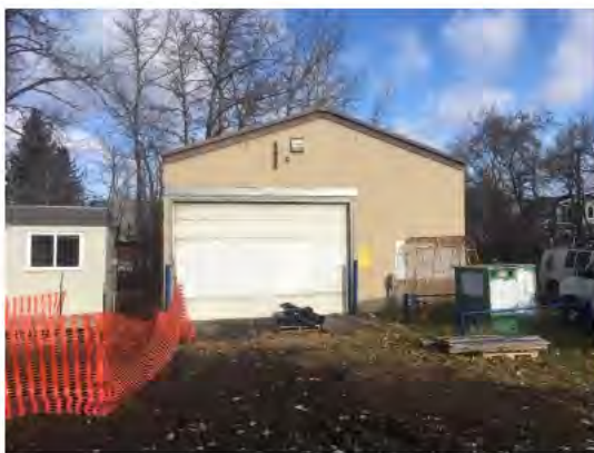
Garage located east of the new trailer.
