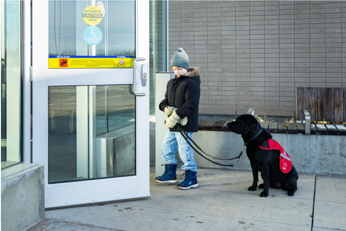
Image B.1(a) An accessible building entrance
