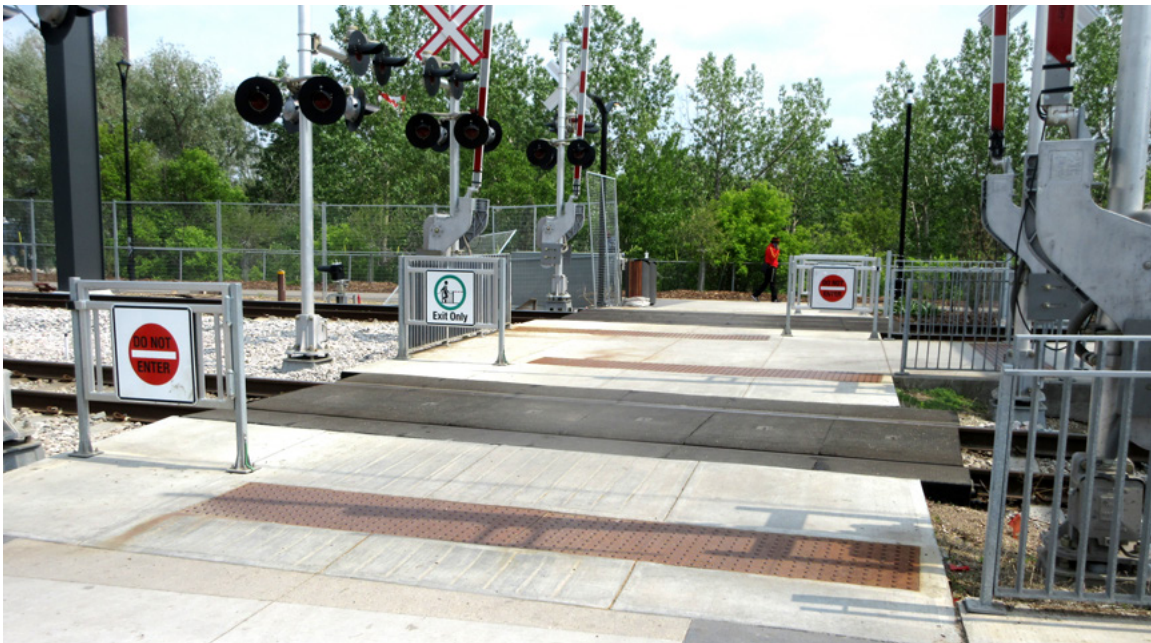
Image A.4.1(b) Pedestrian path at rail crossing
