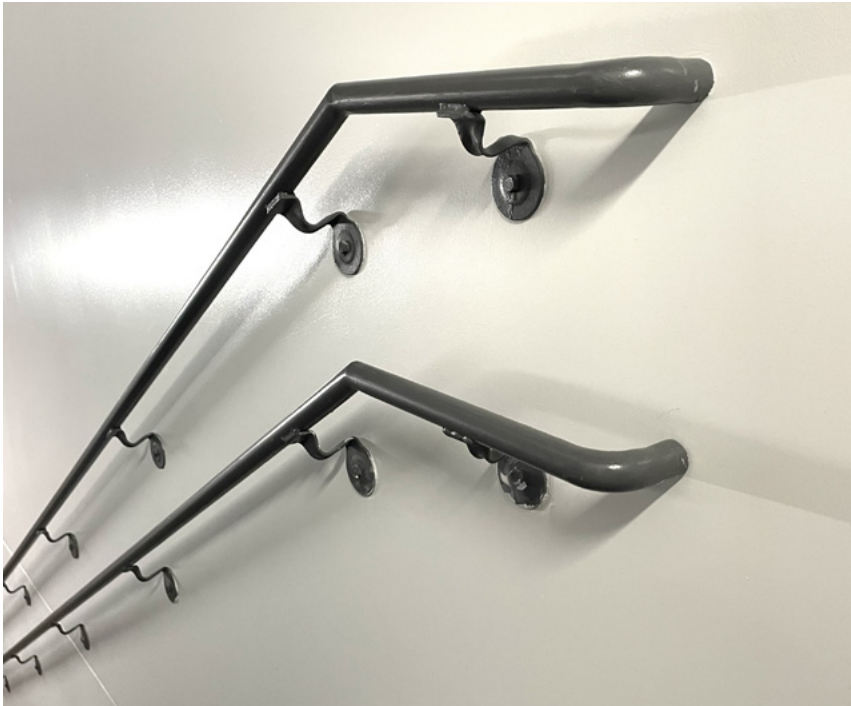
Image B.2.1.5(b) Additional handrail at lower height
