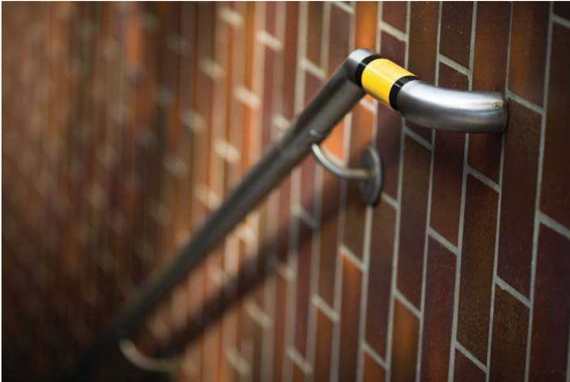
Image B.2.1.5(a) (Source: Clearing our Path Version 2.0 ) Luminance contrasting strip on handrail
