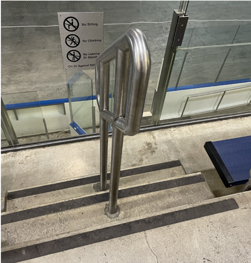
Image B.2.3.3(a) Contrasting strips on aisle steps
