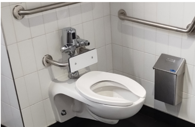
Image B.2.5.3.3(a) Back support for water-closet users
