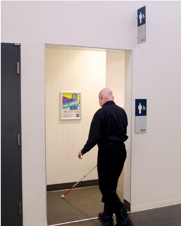
Image B.2.5.3.1(a) Doorless washroom entrance
