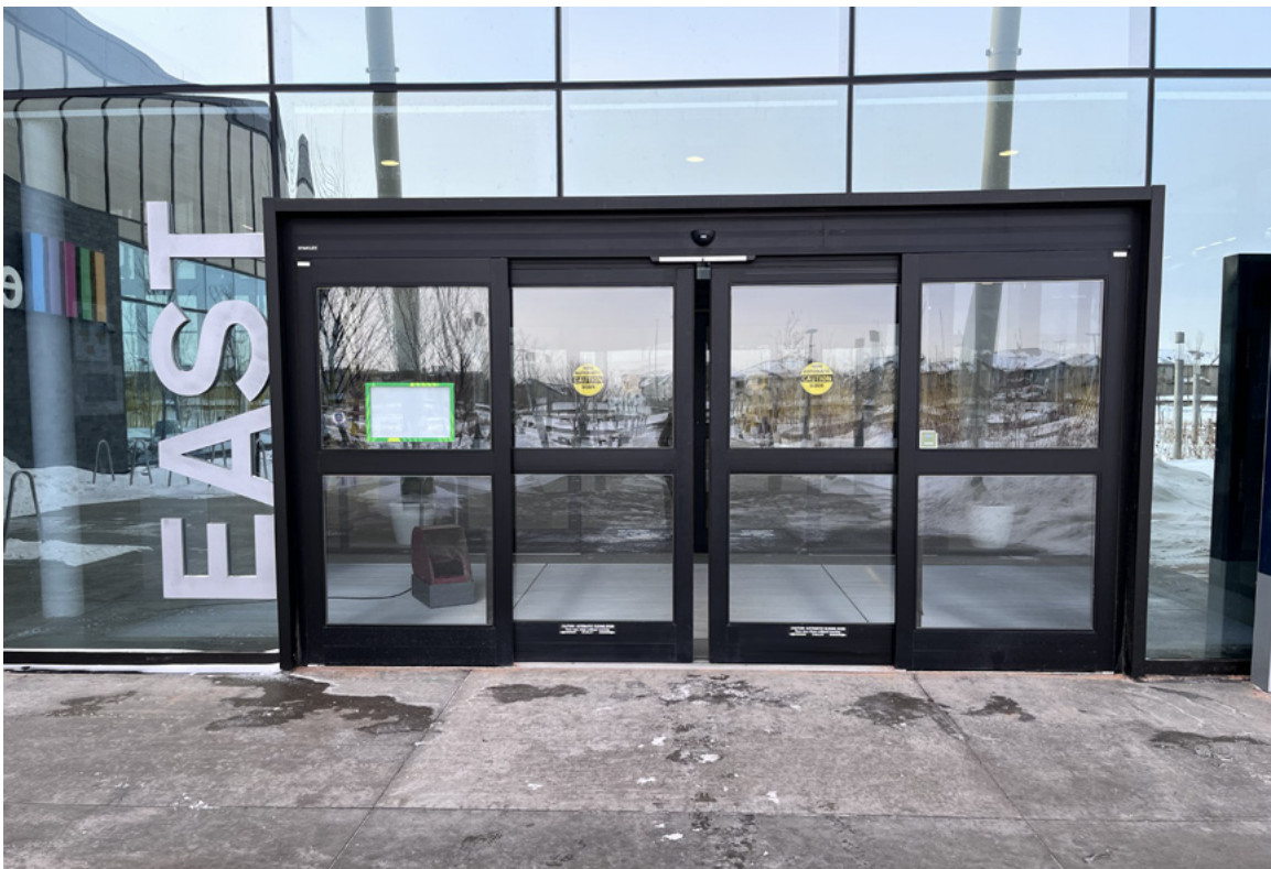
Image B.1.1(a) Clearly marked entrance doors
