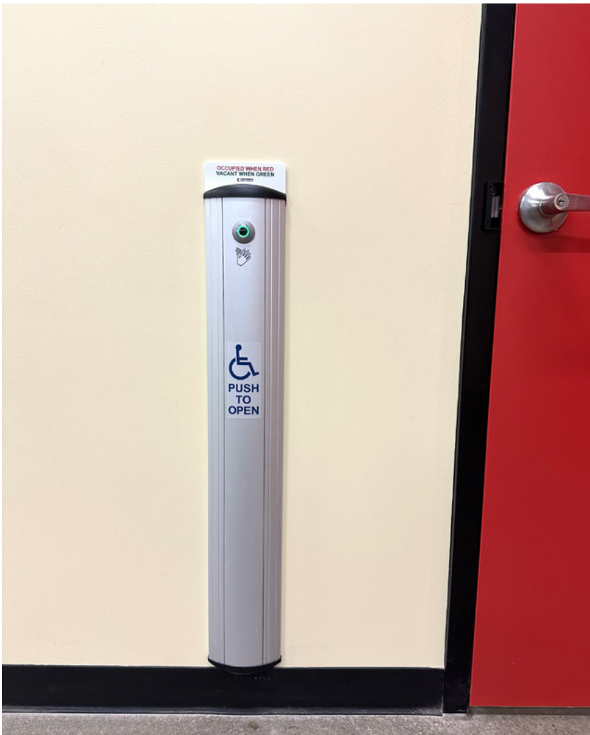
Image B.1.1(b) Push plate with integrated touchless sensor
