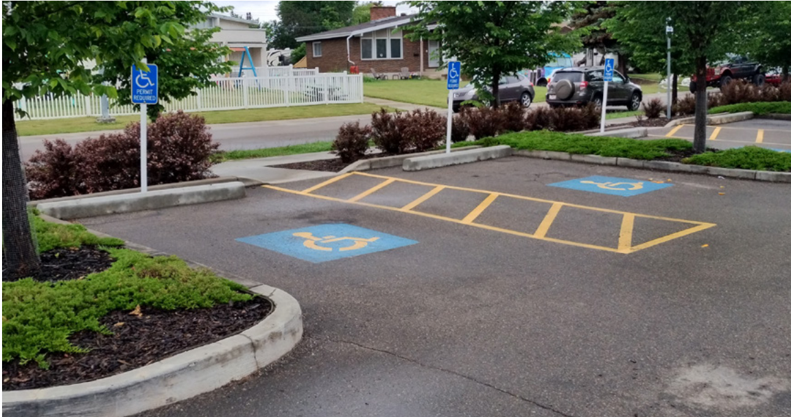
Image A.5.2.2(a) Off-Street Accessible Parking Stalls
