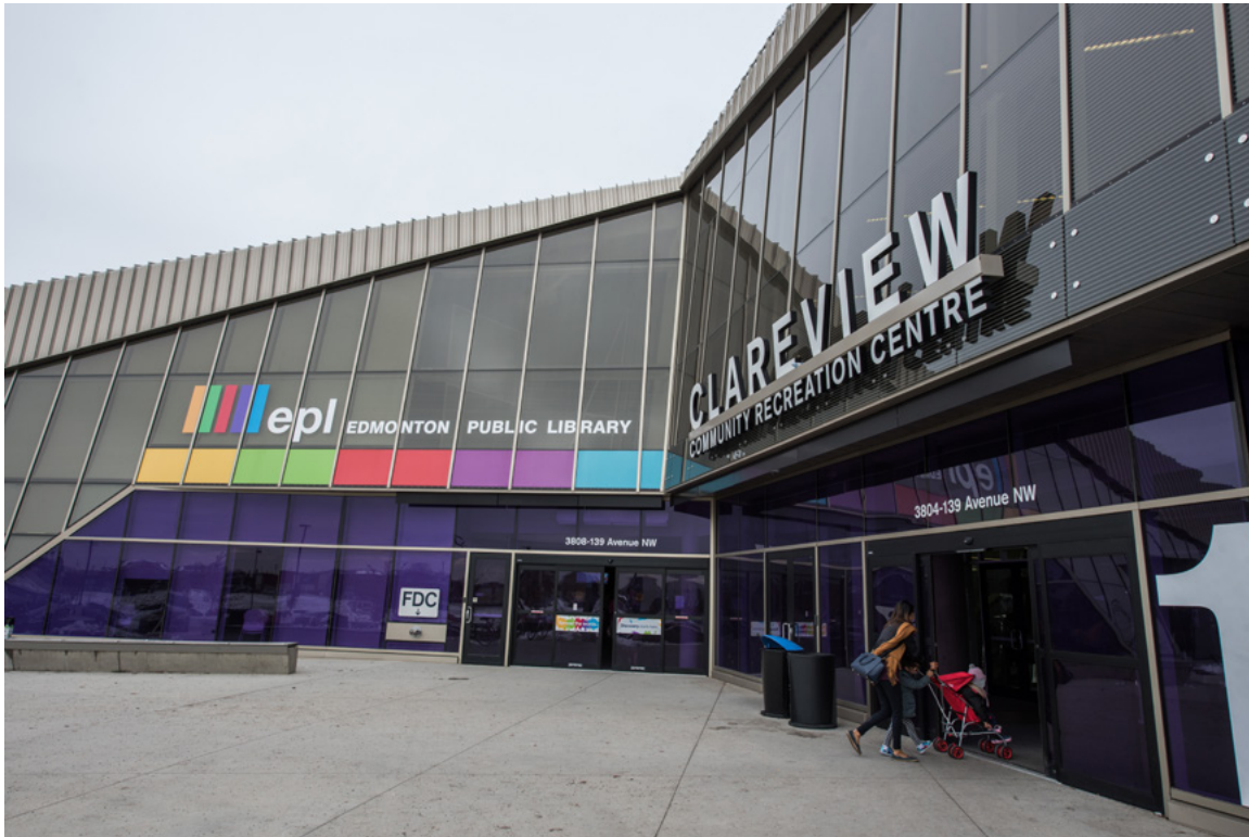
Image B.3.1(a) Exterior building identification sign
