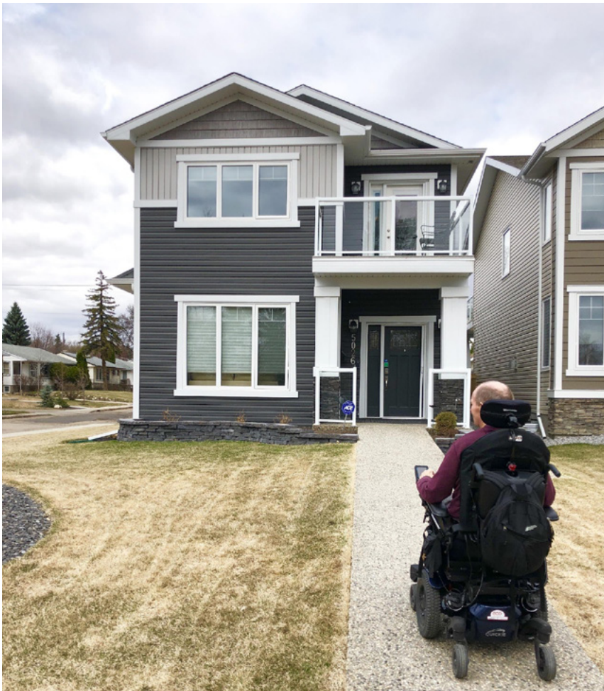
Image C.1.1(a) Accessible front entrance
